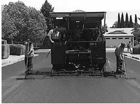
Pavement preservation treatments for asphalt pavements can include slurry seals, which are shown here.
