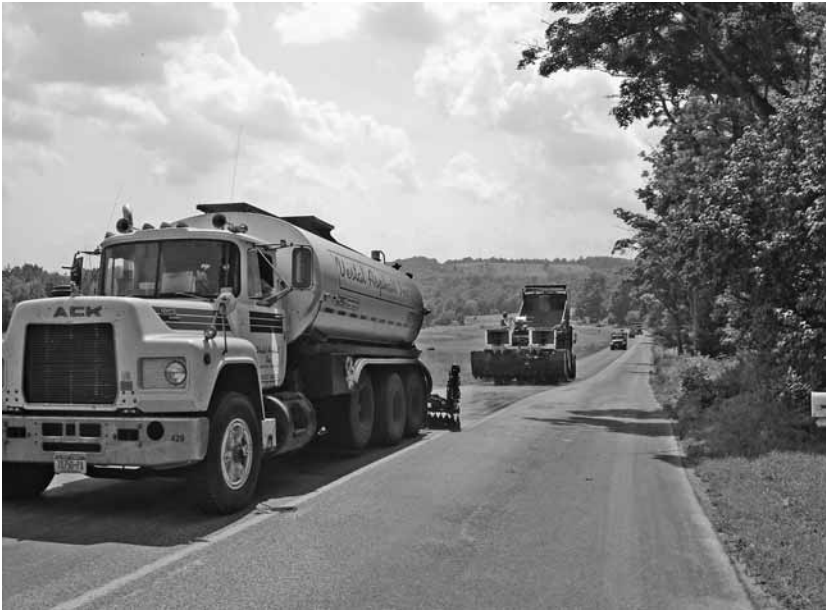
The chip seal program has been a mainstay in Delaware County's maintenance approach to keep roads in good serviceability.
