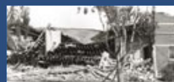
These are the remains of Jefferson Junior High in Long Beach, Calif., following the earthquake on March 10, 1933.
