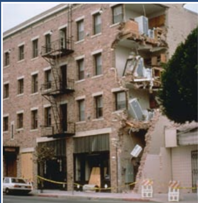
Unreinforced masonry buildings are especially vulnerable during strong earthquake shaking. Shaking-hazard maps are used to determine areas where these types of buildings need to be reinforced to make them safe during earthquakes. Photo: J. Dewey
