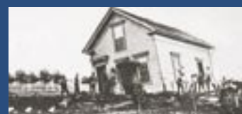
This home was damaged in the magnitude-6.9 earthquake on the Hayward Fault on Nov. 21, 1868.
