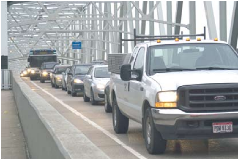
Taylor Southgate Bridge connecting Cincinnati, OH and Newport, KY.
