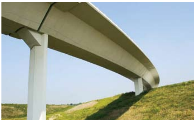
The I-70 ramp west of Indianapolis, a Fast Track project. Photo courtesy of INDOT.
