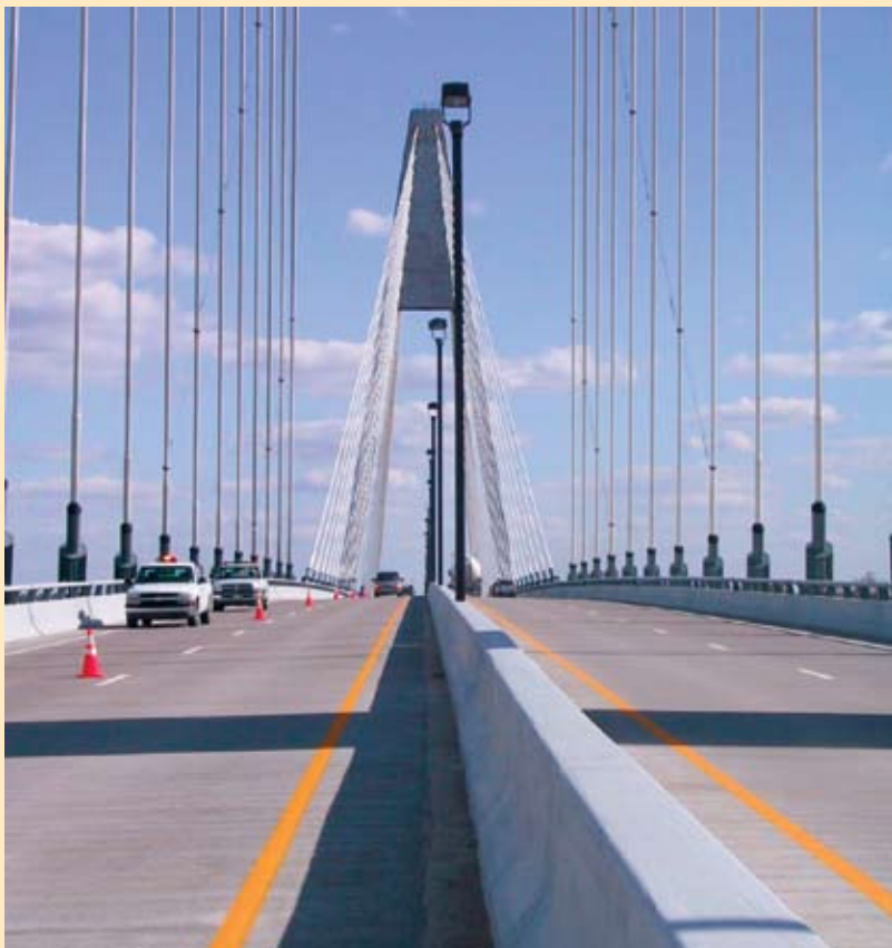
Work on the Ohio River Bridge on US 231. Photo courtesy of INDOT Bridge Section.
