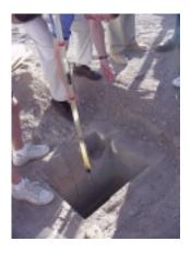
a. Regular monitoring of the sludge and scum layers in all chambers of the septic tank. The septic tank should be pumped when the thickness of the sludge layer and the scum layer exceeds 1/3 of the septic tank's total height. Failure to pump a septic system will result in solids flowing out to the drainfield, which will clog the soil pores and cause drainfield failure.
