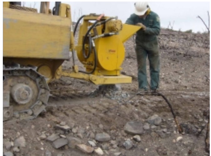
Figure 6—Feeding rocks into the crusher; dozer is stationary.
