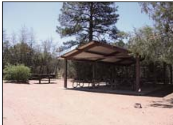
Figure 16–18—The accessible group gathering area has a shelter, group-sized pedestal grills, a serving table, and a large fire ring.
