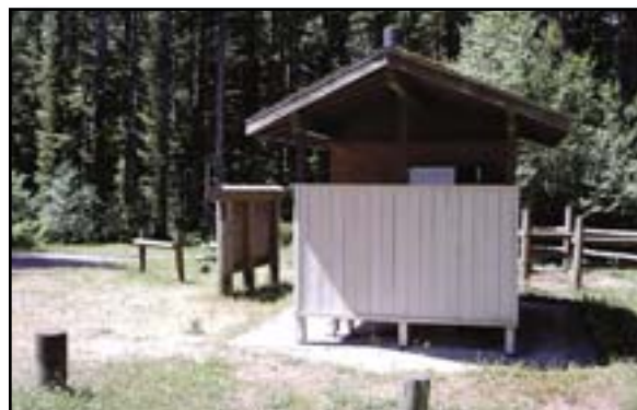
Figure 16-3—Members of the Job Corps built the sturdy vault toilet.
