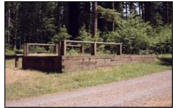
Figure 16-6—A combination mounting and loading ramp is provided for people who use mobility devices and for trail stock.
