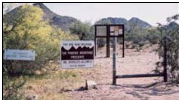
Figure 10-19—As heavy traffic wears the tread down, negotiating stepovers may become more difficult for all users. This trail gate is not accessible to people with disabilities because the bar across the opening is higher than 2 inches.
