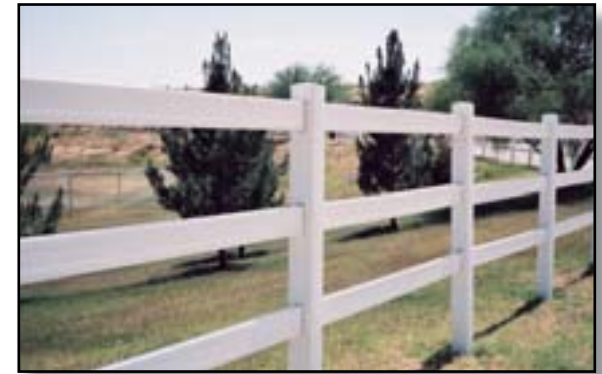
Figure 10-7—When they are installed correctly, vinyl post-and-rail fences are strong, durable, require little maintenance, and have no sharp edges to injure stock.
