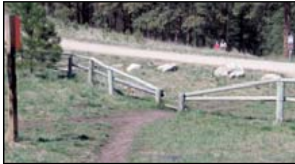
Figure 10-18—Riders, pedestrians, and mountain bikers can pass through this relatively narrow V-gate on a rural trail, but ATVs are restricted. The gate is not accessible to people with disabilities because it is narrower than the minimum width required for passage of a wheelchair—32 inches—and the bar across the opening is higher than 2 inches.
