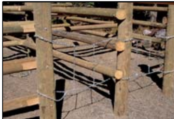
Figure 10–25—Chain gates are simple and effective. Some riders do not like them because a horse or mule may get its head or hoof caught in the large openings.
