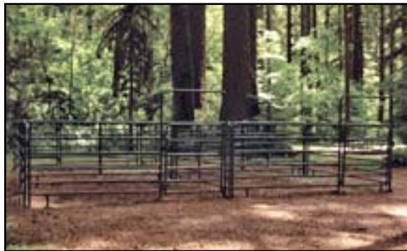
Figure 10–8—Building a corral is quick and easy with premanufactured metal panels.
