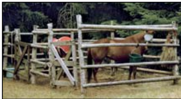
Figure 10–23—Wood corral gates are heavy and can sag over time. This corral has rails attached to the outside of posts. A horse could pop the rails loose by leaning against them.
