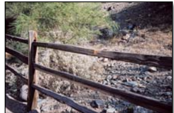
Figure 10–3—Some rustic wood fences have inline rails that pass through holes in the posts.
