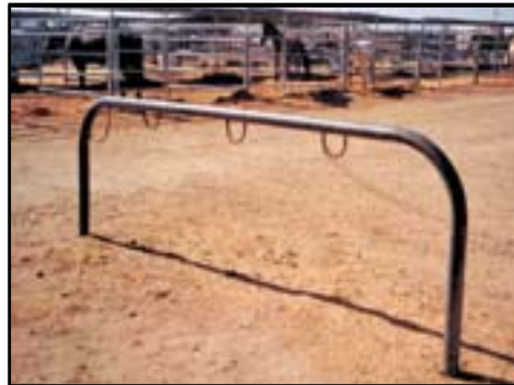
Figure 10–45—Welded steel loops prevent lead ropes from sliding along this hitch rail.
