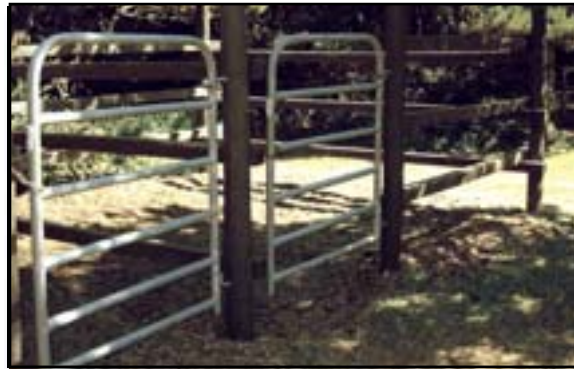
Figure 10–24—Premanufactured tubular steel gates are lighter and less likely to sag than wood gates.
