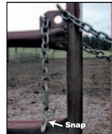
Figure 10-32—Premanufactured gates often come with a slot latch and chain to wrap around the gatepost. Attaching a sturdy snap that can be hooked back into the wrapped chain prevents most curious horses and mules from letting themselves out.
