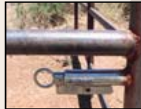
Figure 10-33— This galvanized latch is horse resistant.
