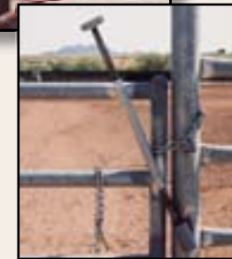
Figure 10-38— Pull-rod latches allow riders to open gates without dismounting.
