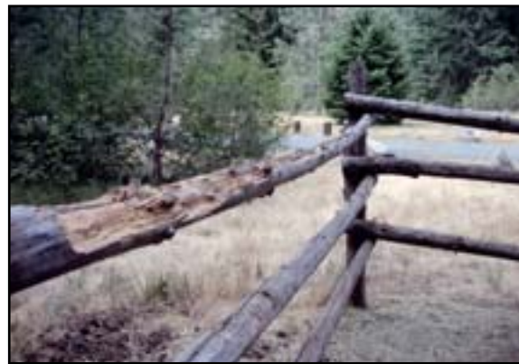
Figure 10–4—Hungry or bored stock often chew on inappropriate items, causing considerable damage.
