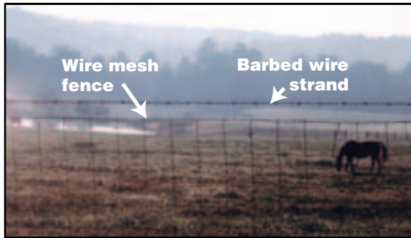
Figure 10-9—Barbed wire discourages cattle from leaning over and breaking down a fence, but can be dangerous for horses and mules. Choose an alternative fencing material in recreation sites.
