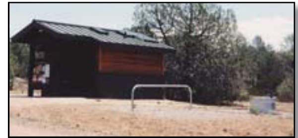
Figure 10-50—Areas near toilet buildings are excellent places to install hitch rails. Provide plenty of clear space around the hitch rails. This rest area also includes a horse trough nearby, a welcome amenity.
