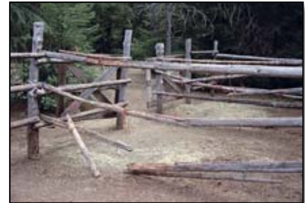
Figure 10–5—Riders repair corrals with whatever materials are available—in this case, baling twine and wire. Schedule regular inspections and maintenance so riders don't have to make repairs themselves.
