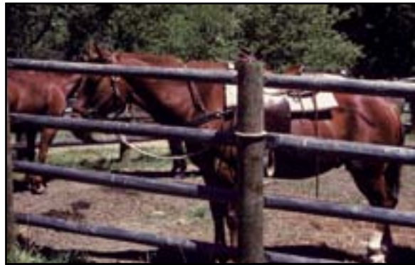
Figure 10-6—Sizable rails, attached to the inside of posts, define a classic wood corral.
