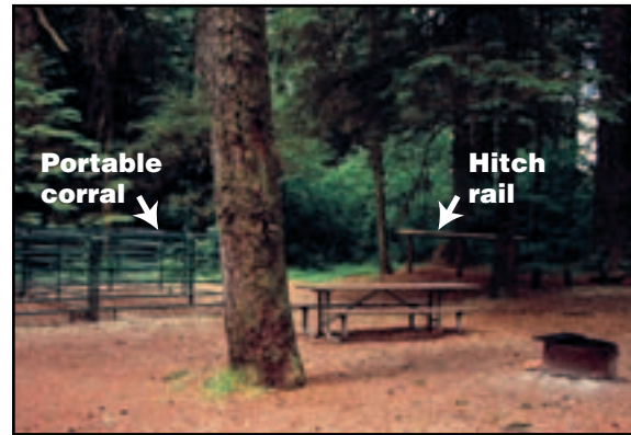
Figure 9–9—Unless they have permanent posts, portable corrals are not strong enough to be used for tying stock. A separate hitch rail is much sturdier and safer.
