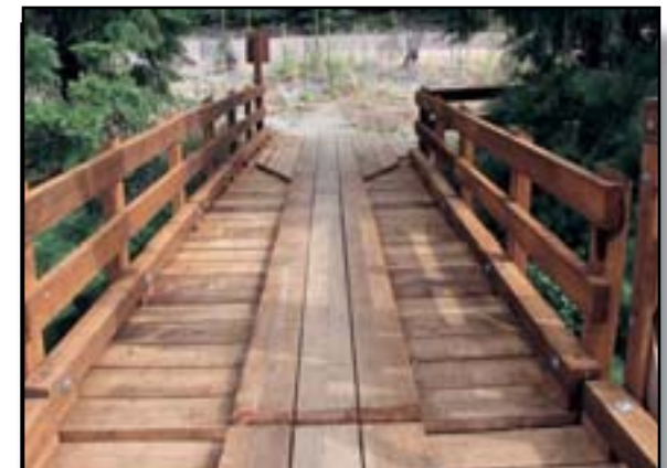
Figure 5-22—Wearing surfaces are a relatively easy and economical way to prolong the life of bridge decking. The tapered pattern guides stock to the wearing surface in the center of the bridge.
