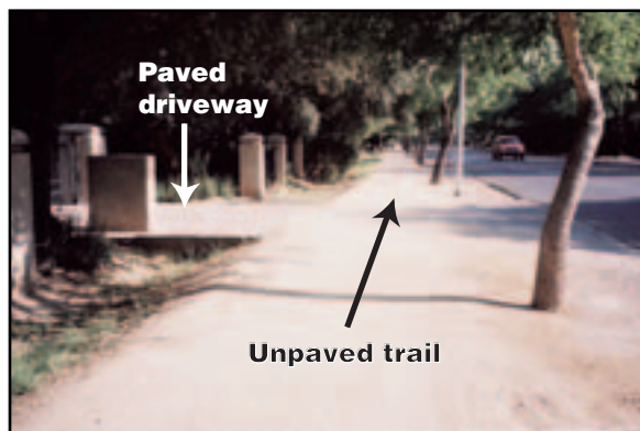
Figure 5–5—Unpaved trails that continue across driveways are more comfortable for riders than trails that are interrupted with pavement. The Murphy Bridle Path in North Central Phoenix, AZ, was established in 1895 and preserved as an unpaved trail in the heart of a modern community. Unpaved trail sections across driveways may not be suitable in all regions of the country.
