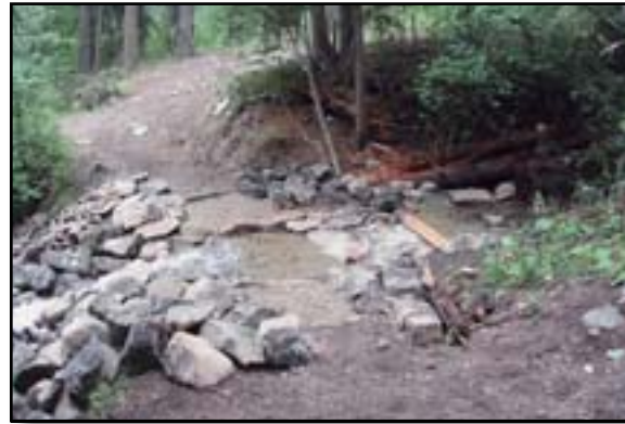
Figure 5-8—This fish ladder includes a ford for trail users while still allowing trout to move up the creek. The steps have big landings—about 8 to 10 feet long—and stock tolerate them. The rocks alongside the ford keep stock on the desired path.
