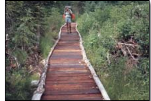
Figure 5–16—Puncheon walkways can be level with the surface or lie below it. Log stringers support this deck.
