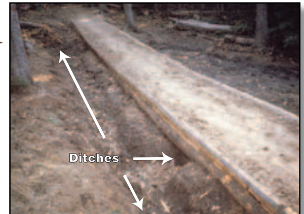
Figure 5-15—A turnpike elevates the trail in boggy or wet areas. Ditches provide drainage. This turnpike has log stringers filled with coarse, well-drained rock.
