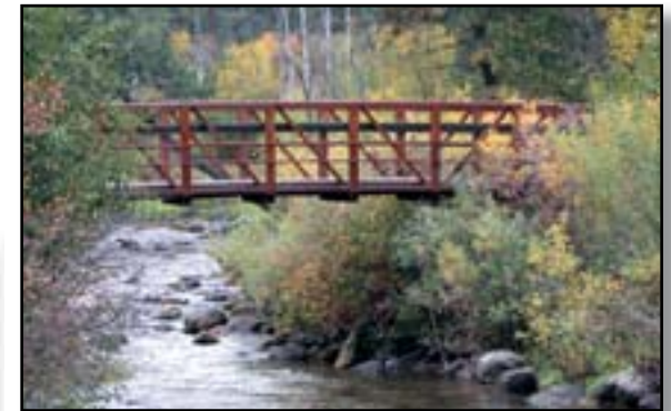
Figure 5–18—The weathered steel and wood of this sturdy stock bridge fit the setting.
