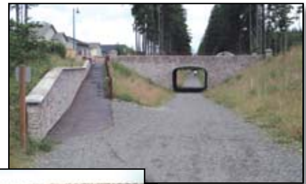
Figure 5-30—Make horizontal trail clearance in underpasses the same width as the trail or wider. — Courtesy of Bridgetek.
