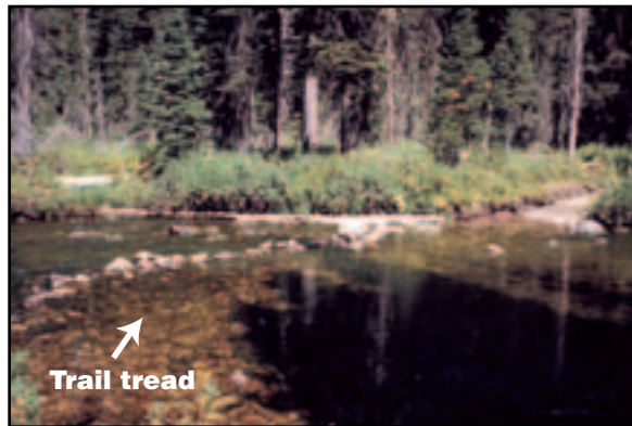
Figure 5-12—A stable tread surface is essential for shallow stream crossings. Stepping stones for pedestrians should be placed on the upstream side of the tread.
