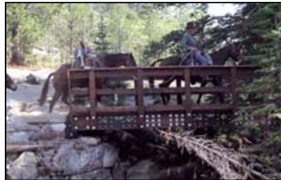
Figure 5–17—This packable bridge comes in 6-foot sections that are bolted together at the site. Nearby cliffs encourage stock to stay on the tread, so approach rails are unnecessary.
