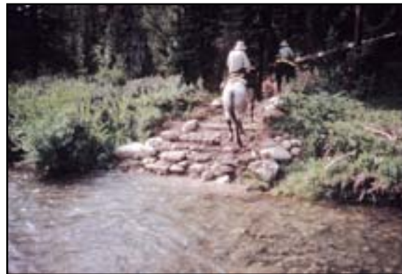
Figure 5-13—Rocks and gravel can be used to reduce erosion along waterways, but medium and large rocks can be slippery when wet. These riders chose the side of the tread with the best horse footing—small rocks and gravel.
