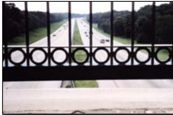
Figure 5-23—A solid barrier topped with an open view railing is often more acceptable to horses and mules than an open view fence alone. This open view railing is on the Marjorie Harris Carr Cross Florida Greenway Land Bridge. Figures 5-27 and 5-28 show additional views of the land bridge.
