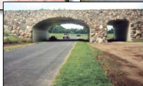
Figure 5-31—For safety, provide separate underpass routes for motorized users and trail users. — Courtesy of Bridgetek.
