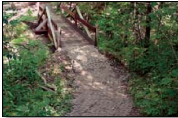
Figure 5-11—The approach to this trail bridge is reinforced with interlocking pavers to withstand wear from off-highway vehicle use. The pavers may not offer enough traction for horses and mules. A similar approach using horse-friendly pavers could be used on equestrian bridges.
