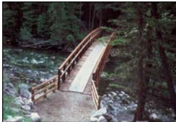
Figure 5-24—Approach rails guide stock onto a bridge. Large rocks or other natural objects sometimes are used to block alternate routes.
