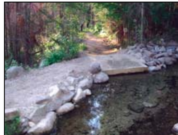
Figure 4–11—After fording the irrigation ditch, stock must step up about 12 inches. Because the landing is only 4 feet square, some untrained stock balk at the step.
