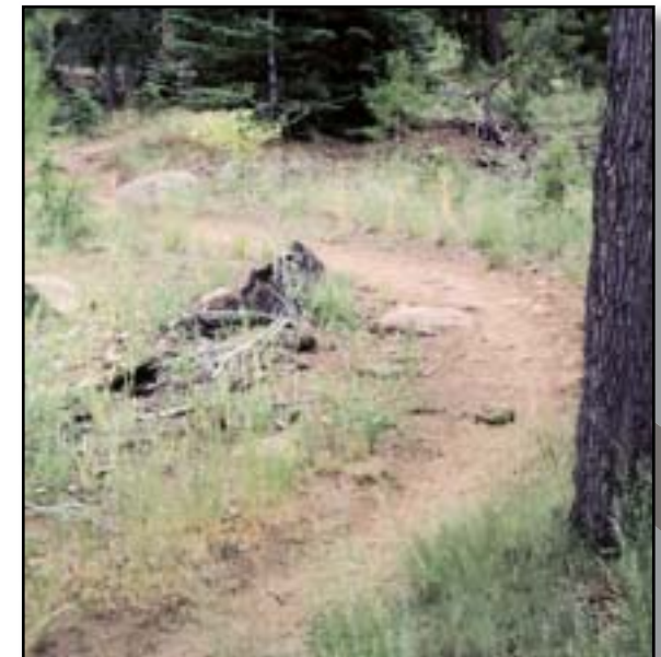
Figure 4–23—Several stumps discourage trail users from cutting across this climbing turn.
