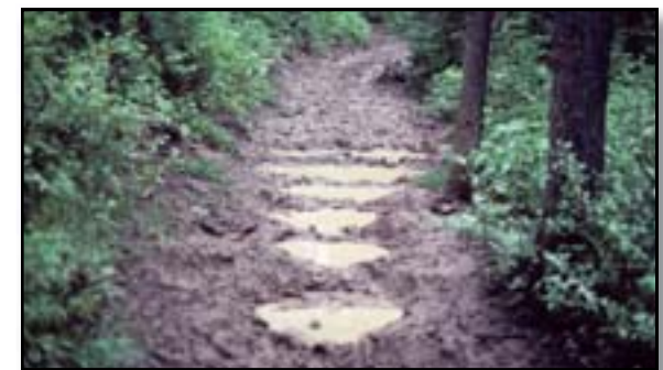
Figure 4-15—Running or standing water can cause extensive damage.
