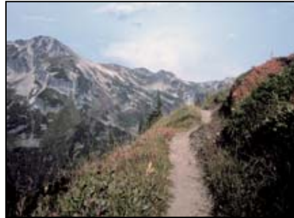
Figure 4–8—Elevation on contour trails remains relatively constant. Trail users appreciate contour trails because they are easier to travel and frequently offer great views.
