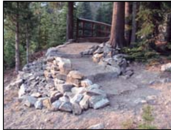
Figure 4–10—Experienced trail stock readily travel these steps to a bridge crossing. The risers are 8 to 12 inches tall, and the landings are 6 to 8 feet deep. The trail tread is about 3 feet wide. Trees and rocks along the sides direct stock onto the bridge.
