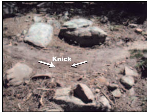
Figure 4-17—A trail knick directs water off relatively flat areas.
