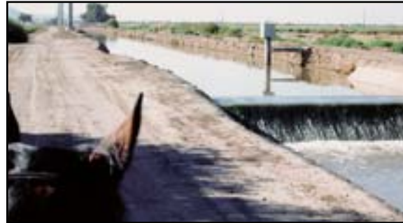
Figure 2–2—Utility maintenance roads are often used for recreation trails.
