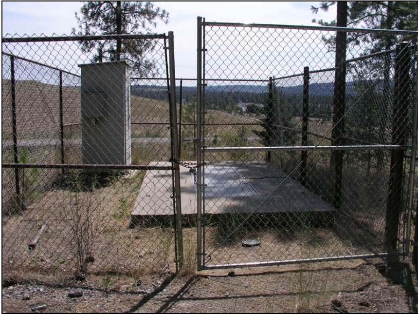
Extraction well (MW-PEW) pump house and power supply
