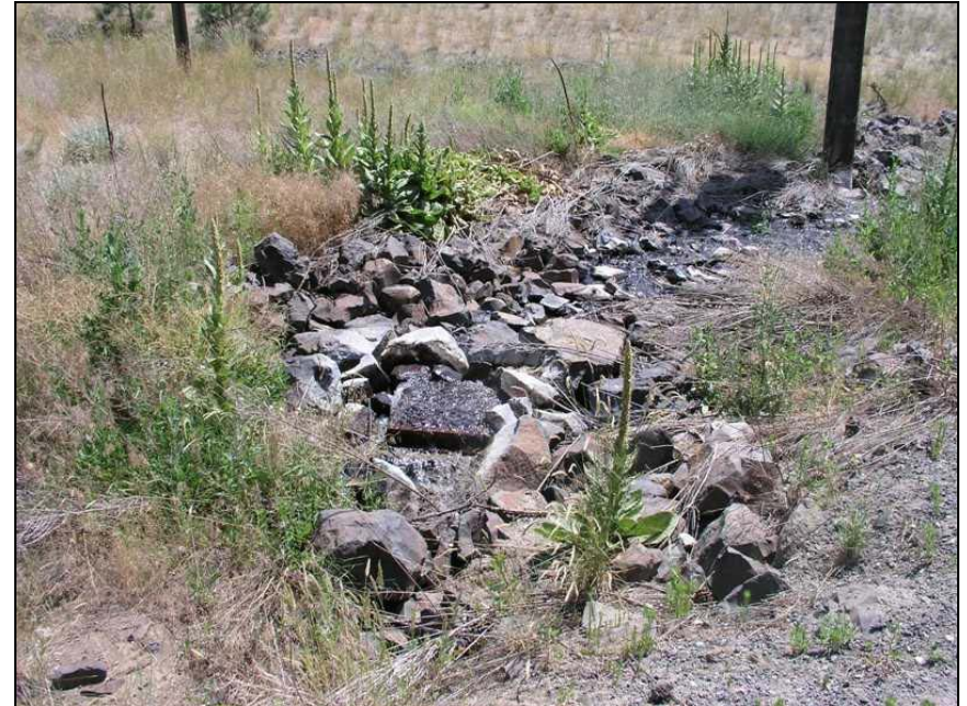
Extraction well outfall
