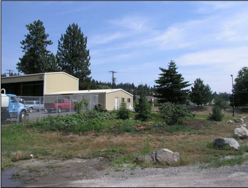
Maintenance buildings, used primarily for active landfill
