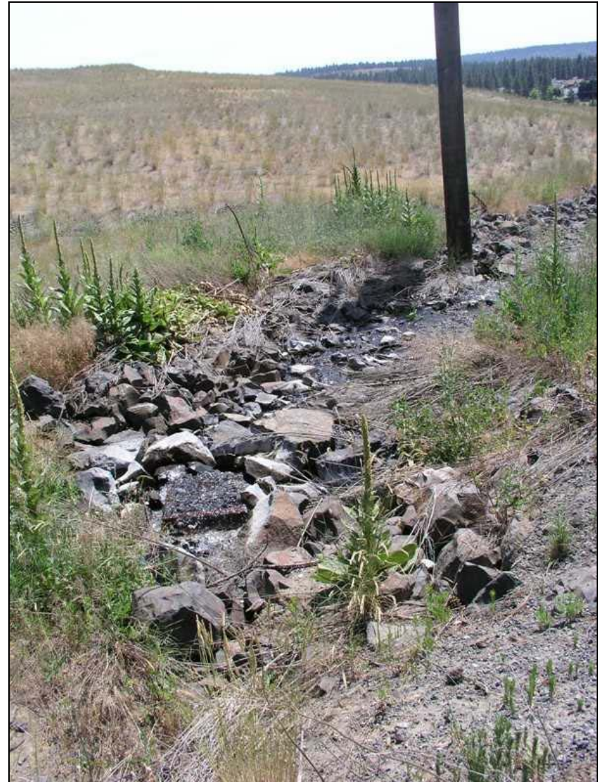
View from extraction well outfall down west side of landfill road (1)
