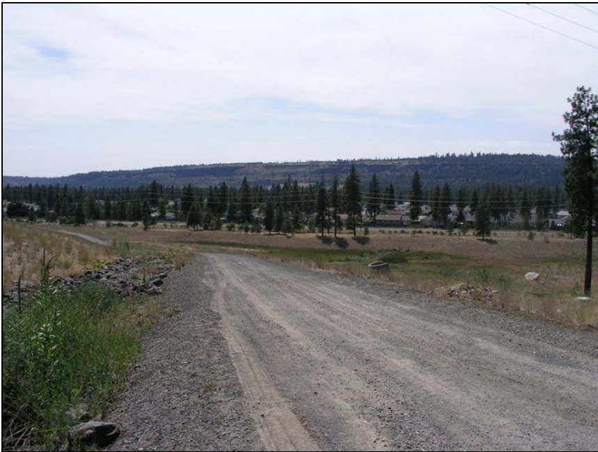
Collection rip rap along road from extraction well outfall to drain
