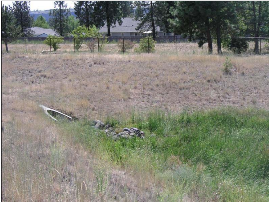
Surface water collection drain on east side of landfill road
