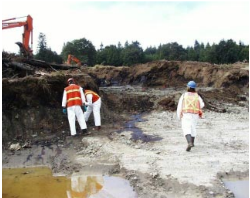
Continuing to excavate the pit, summer 2002
