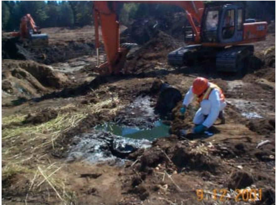
Workers remove buried drums, September 2001
