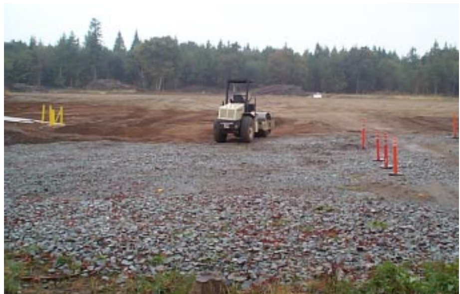
Site after backfill complete, covered with clean soil.
