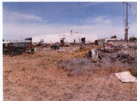
Looking north from the southeast corner of the Stephens Metal Products laydown yard
