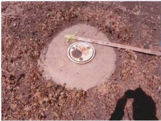
Monitoring well W-14
