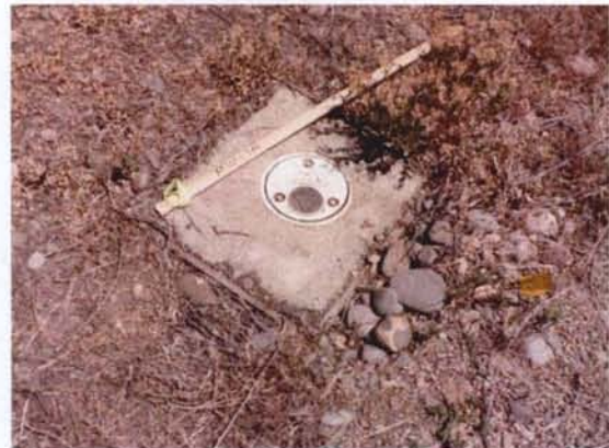
Monitoring well W-18
