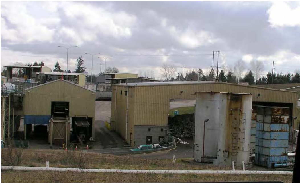
Photo 4: Transfer station and flares.
