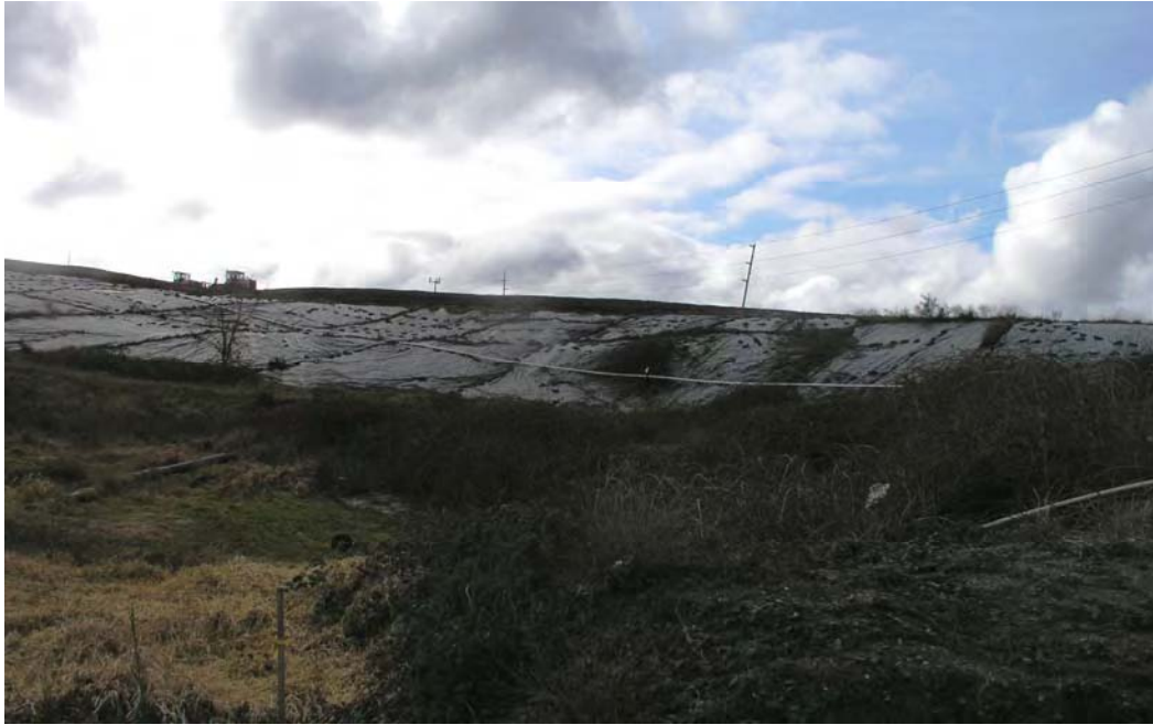
Photo 1: Temporary cap at Central Area.
