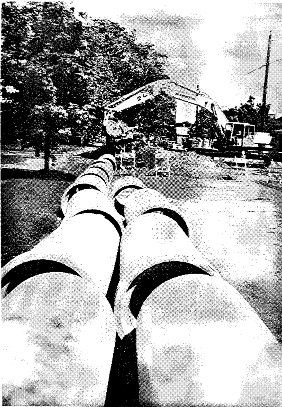
In 1993, 13 miles of new sewer pipe were installed as part of a sewer separation project in Menominee. (Sewer bypassing was also completed in Marinette.) Installation of the pipe eliminated a major combined sewer overflow problem in the area.
