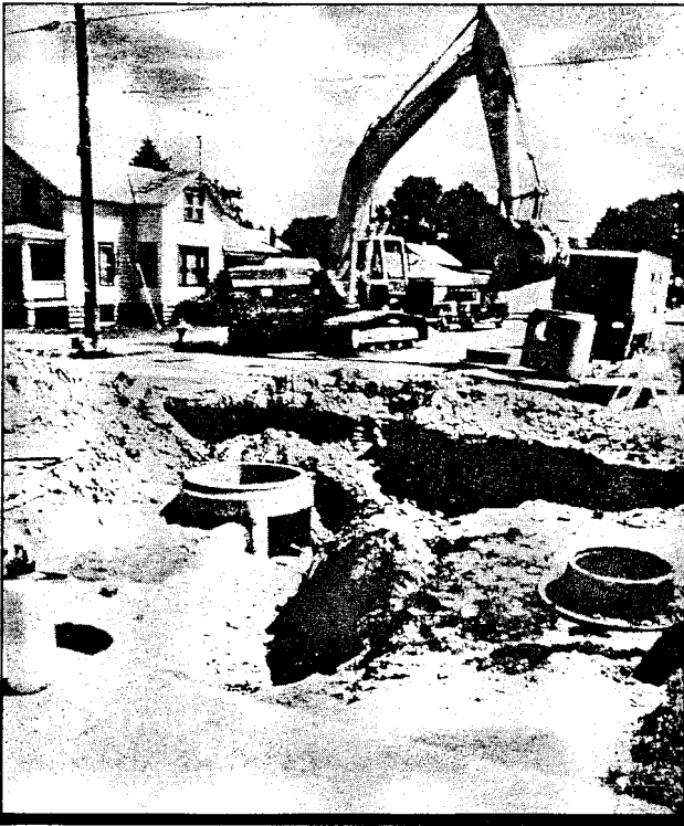
Separation of storm and sanitary sewer systems will help eliminate future discharges of raw sewage into the Menominee River.
