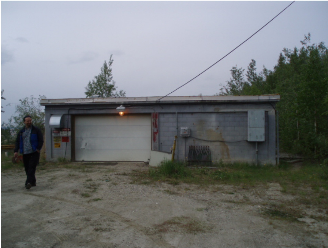
Photograph 13 – Building 1182 (Former Pump House that Contains Product Recovery Equipment), Operable Unit 3
