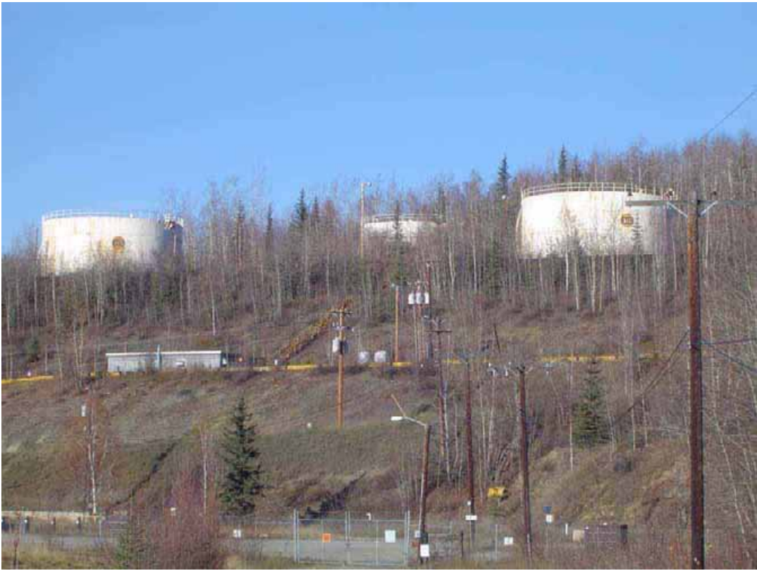
Photograph 11 – View Looking Up at the Birch Hill Tank Farm Operable Unit 3
