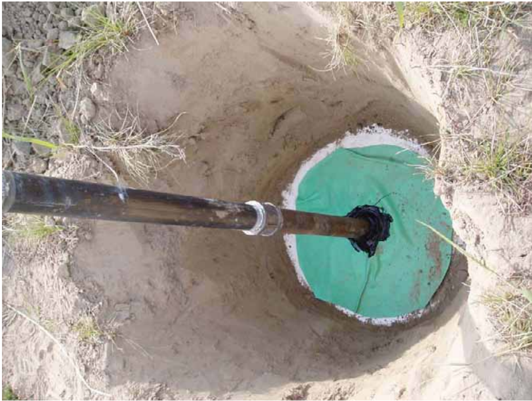
Photograph 3 – Vent Installation, Phytoremediation Cell Operable Unit 1
