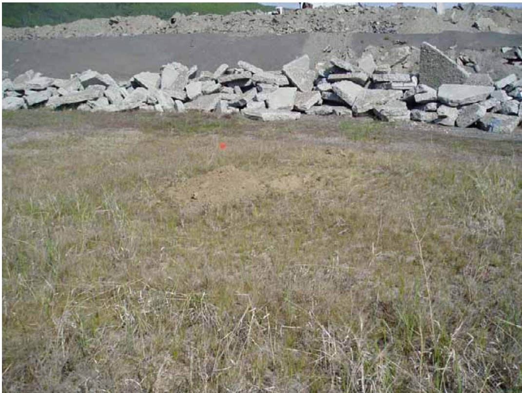
Photograph 2 – Phytoremediation Cell Showing Concrete Berm (flag indicates vent location), Operable Unit 1
