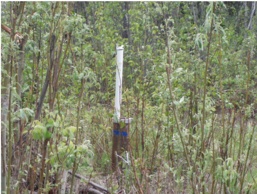
Photograph 20 – Typical Frostjacking of Monitoring Well at Milepost 2.7 & 3.0 Areas Operable Unit 3
