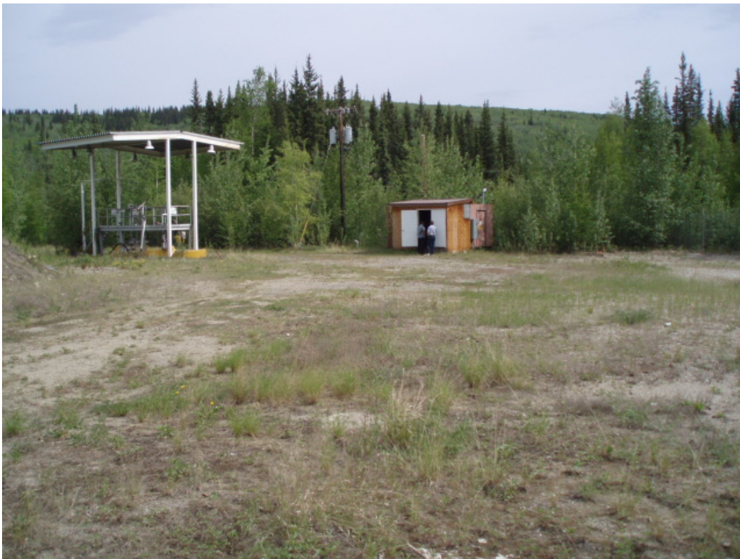
Photograph 14 – Truck Fill Stand and Thaw Channel Treatment System, Operable Unit 3
