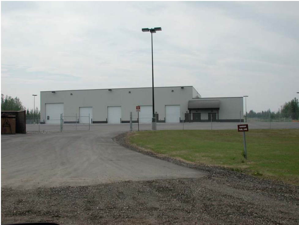
Photo 6: Munitions storage facility constructed at LF03.
