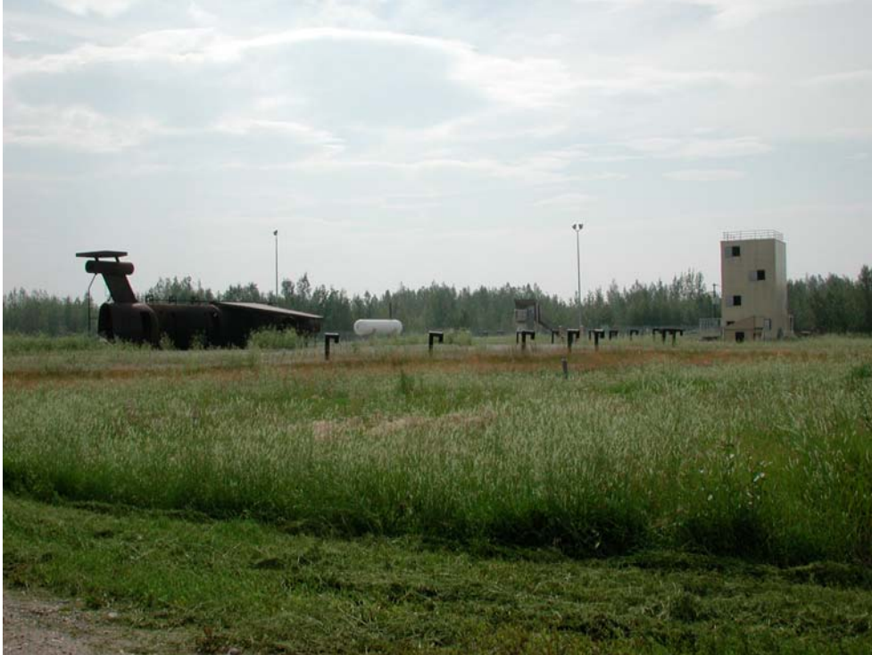
Photo 5: Fire Training Facility at FT09.
