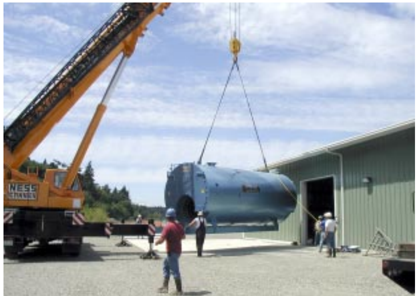
Boiler for steam injection pilot project arrives on-site at Wyckoff/Eagle Harbor.
