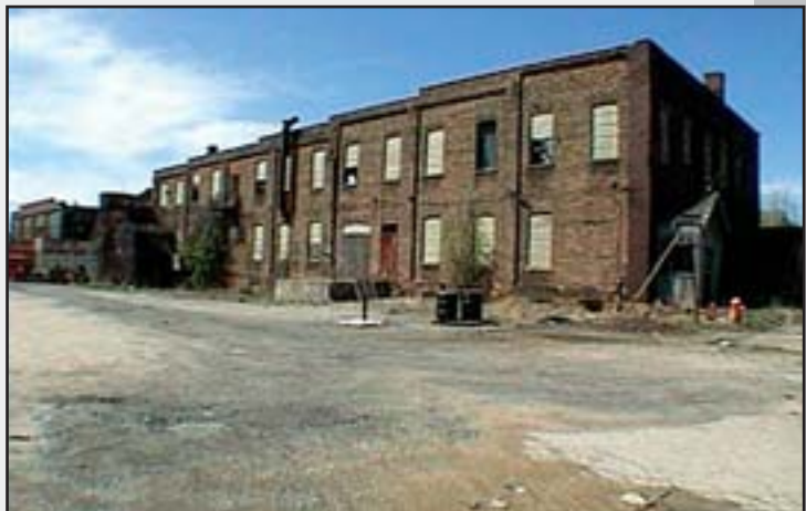
The Wallace Street Foundry Building before renovation.
