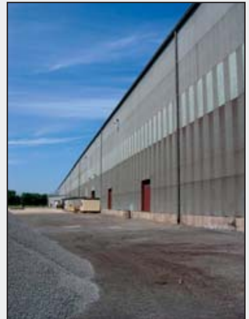
Exterior of the former 14 Inch Mill in Sterling, Illinois, now the Sterling Industrial Park.
