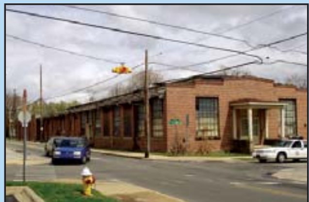
The Grey Hosiery Mill building before redevelopment.
