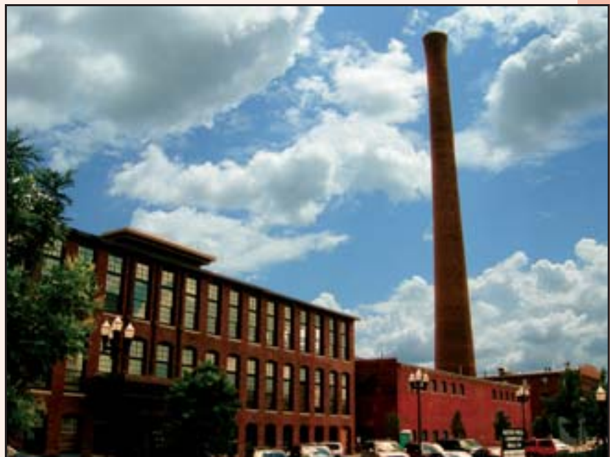
The redeveloped Bates Mill complex in Lewiston, Maine.
