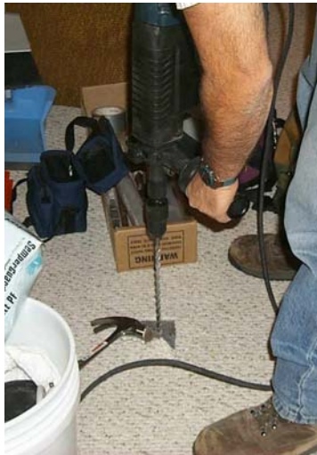
Figure 1. Drilling through slab
