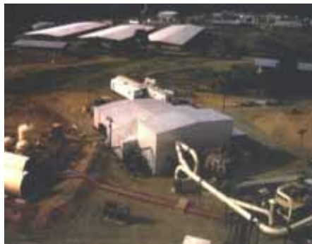
Vertac site incineration facility, Jacksonville, Arkansas.
