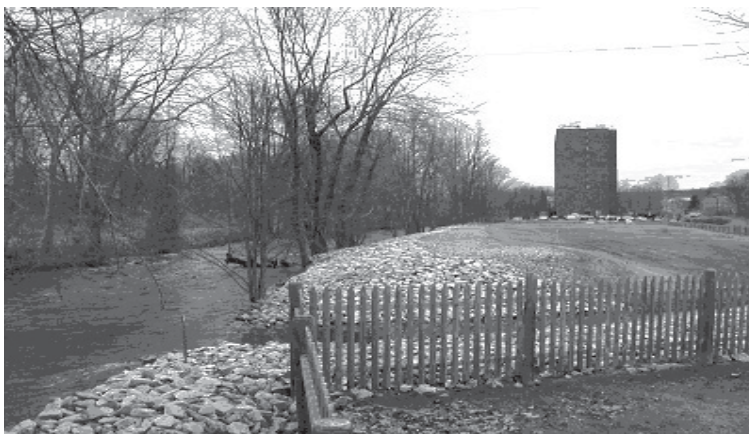
View of the Centredale Manor Restoration Project looking North along the Woonasquatucket River.
