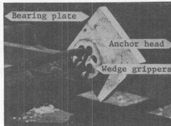
Figure 68. Strand anchorage.
