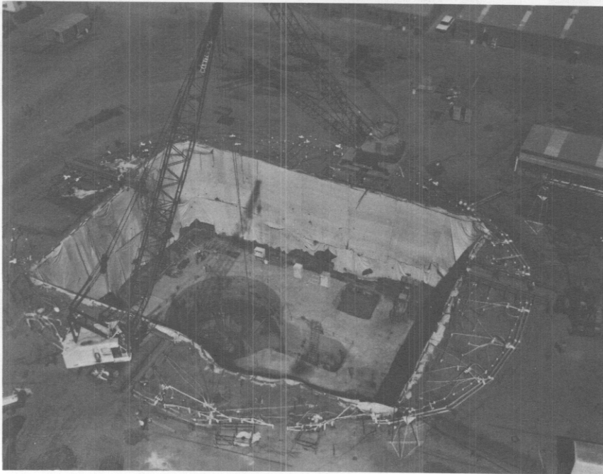
Figure 139. Aerial view of freeze wall surrounding deep excavation.
