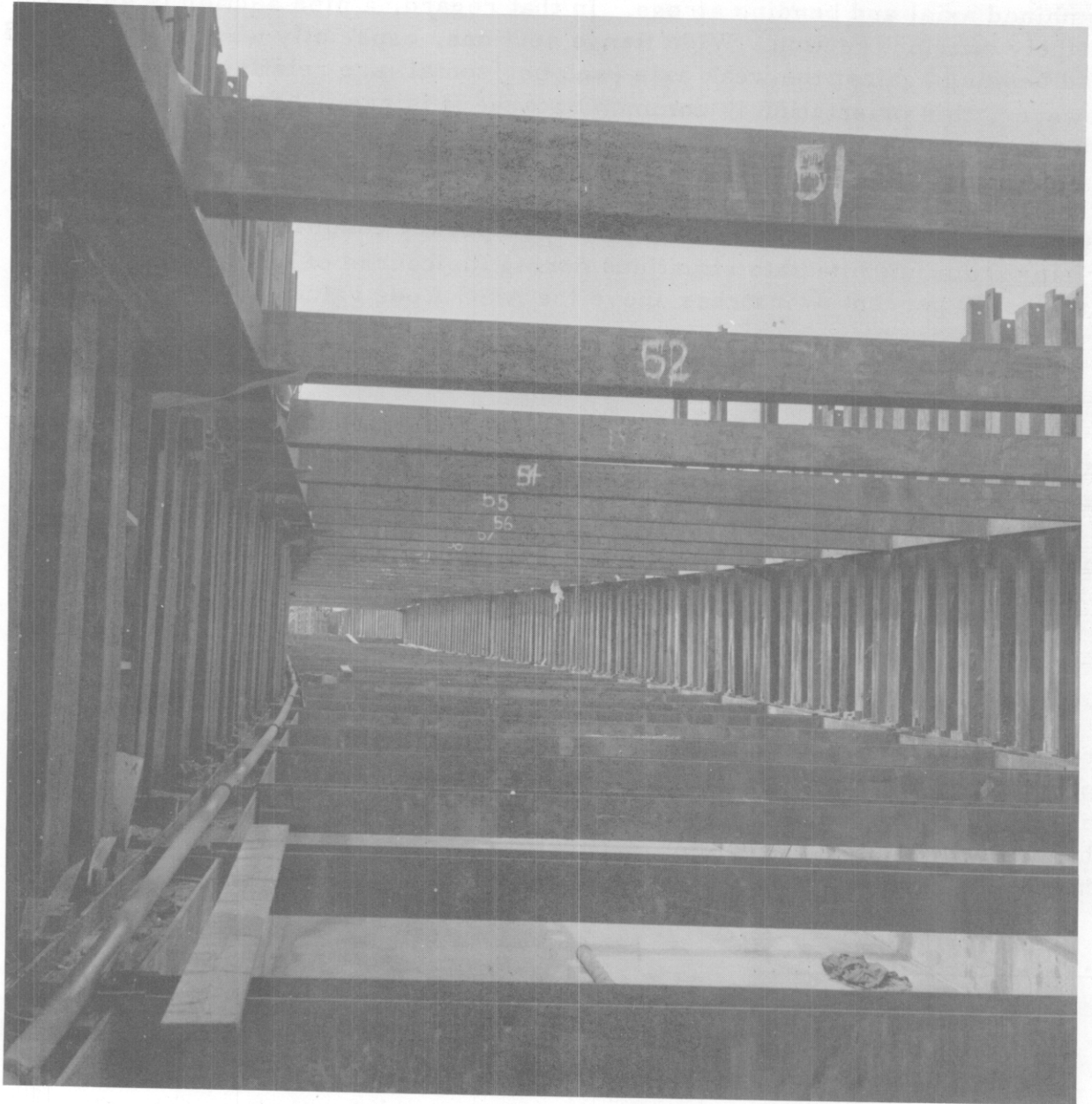
Figure 42. Internal bracing. (Courtesy of Perini Corporation).
