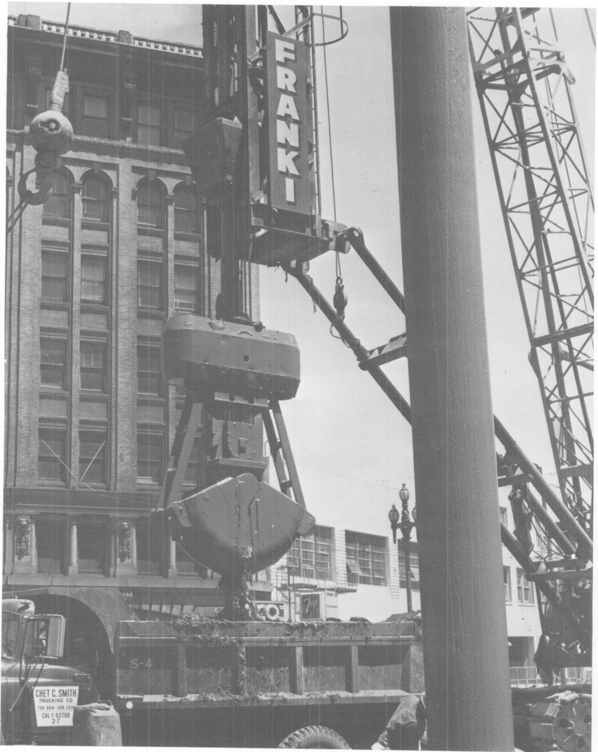
Figure 32. Kelly bar suspended grab. (Courtesy of Franki Foundation).
