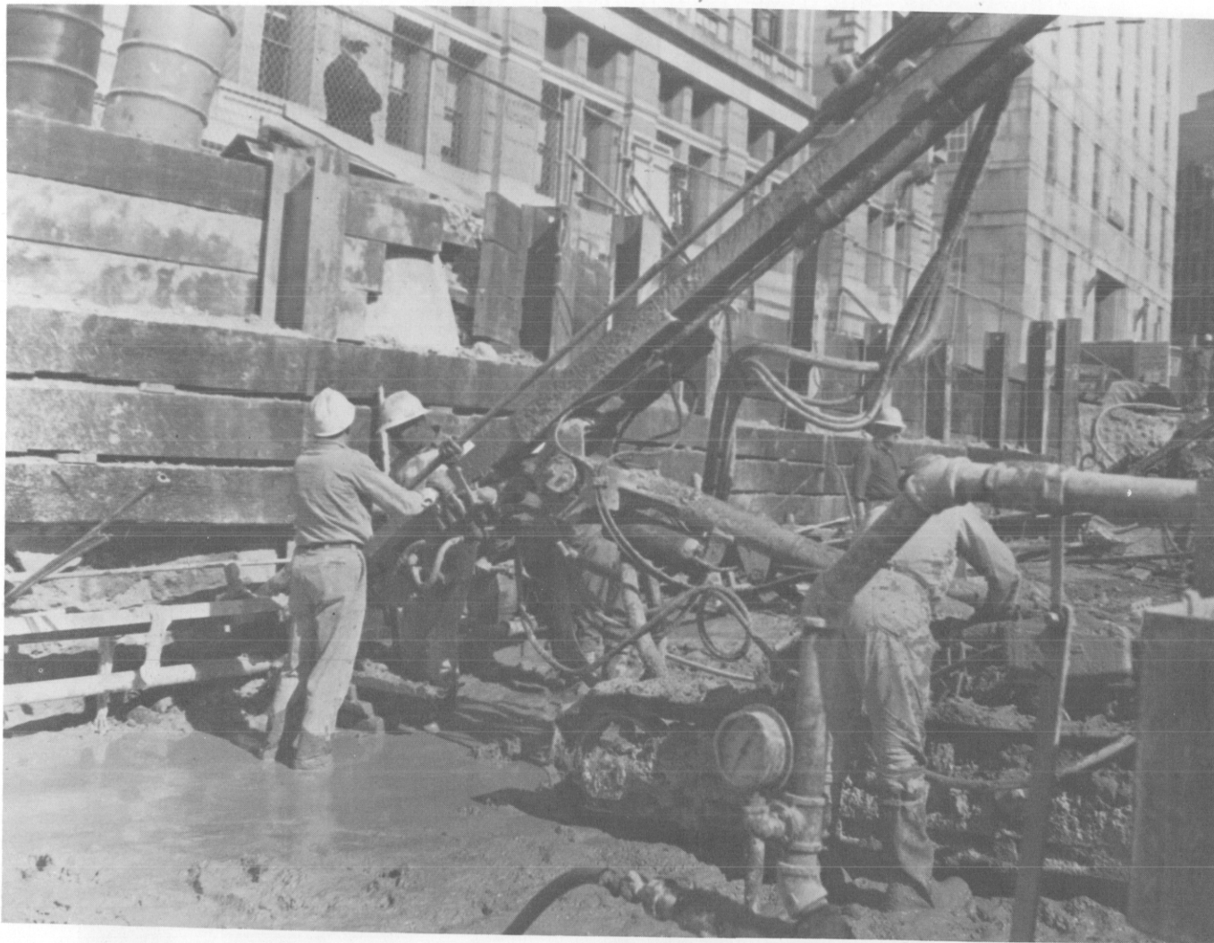
Figure 88. Air trac drilling tiebacks. (Courtesy of Spencer, White, and Prentis).
