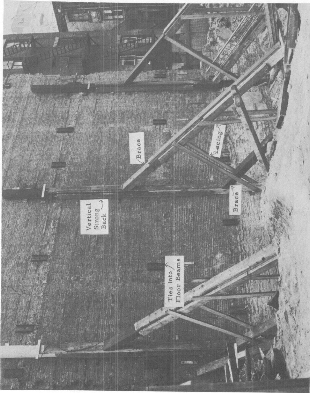
Figure 124. Lateral bracing of wall prior to underpinning. (Courtesy of Spencer, White, and Prentis).
