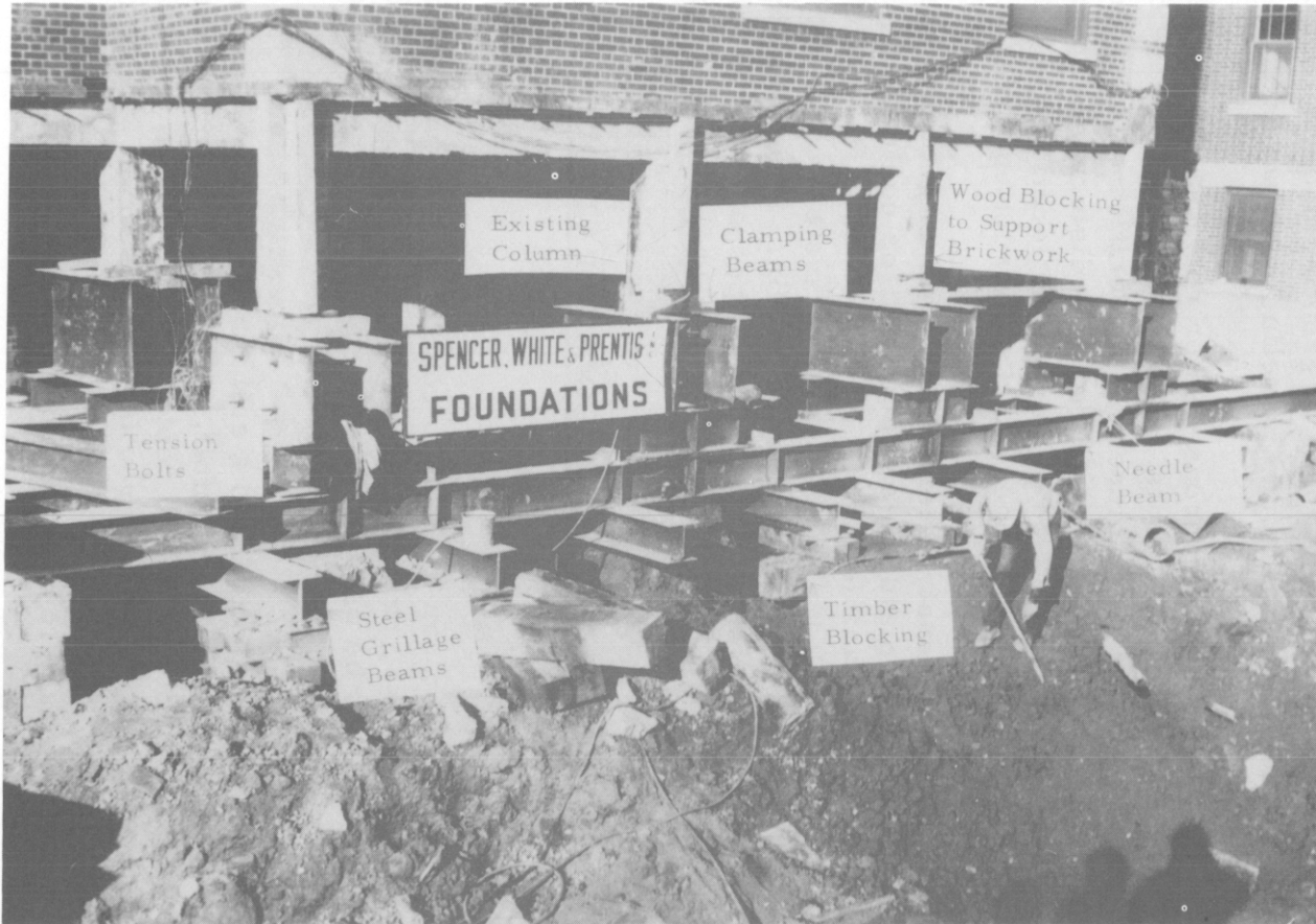
Figure 131. Shoring of concrete columns. (Courtesy of Spencer, White, and Prentis).
