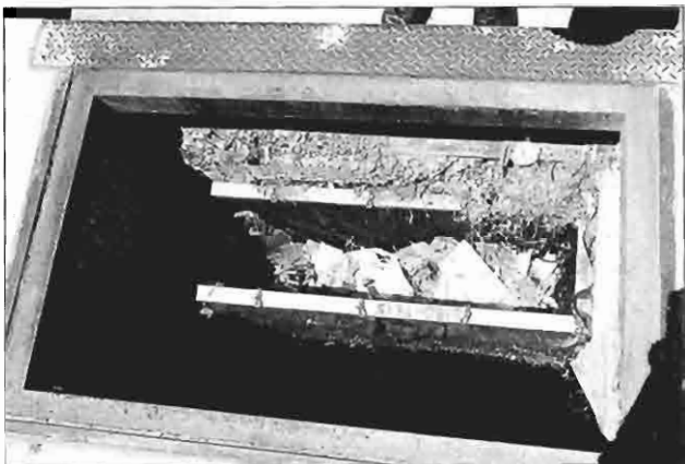
Example of a highway litter monitoring basin
