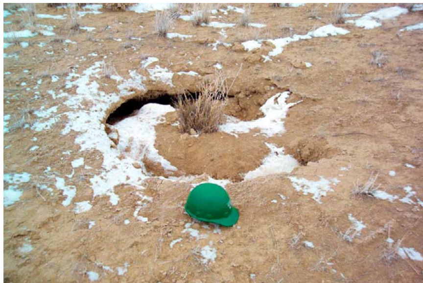
Figure 7-2. Subsidence discovered in the Central Facilities Area Landfill III cover.
