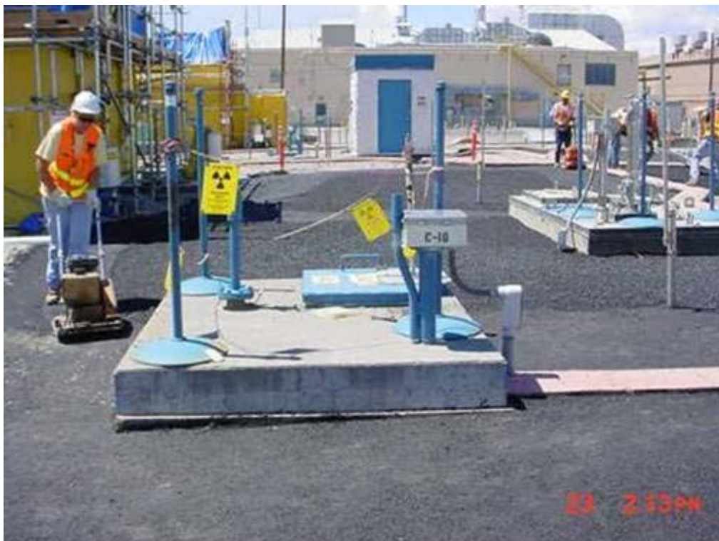
Figure 6-2. Paving activities within the tank farm.
