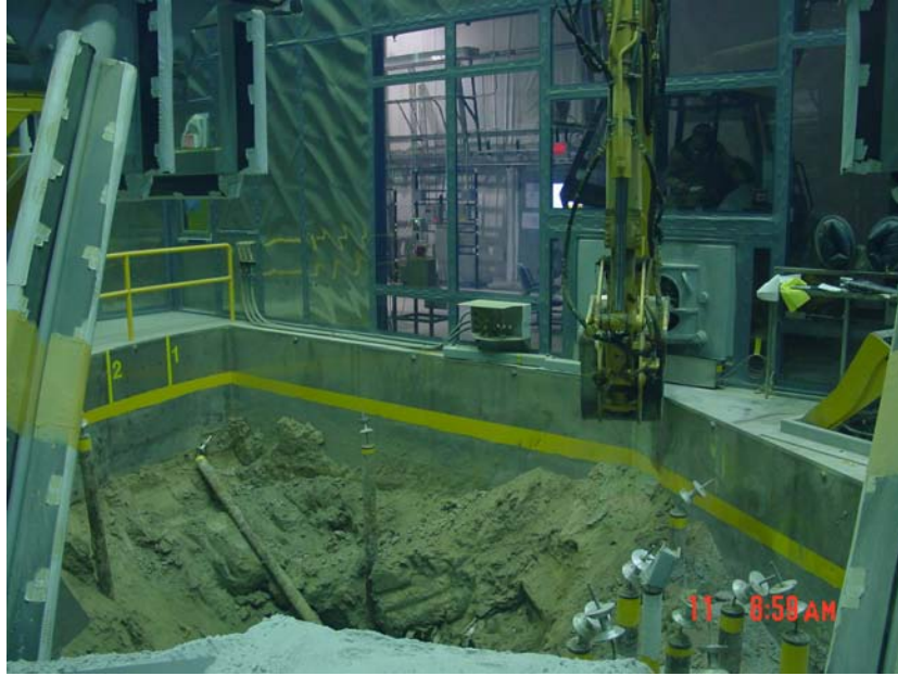
Figure 10-15. The glovebox excavator retrieving waste from Pit 9.
