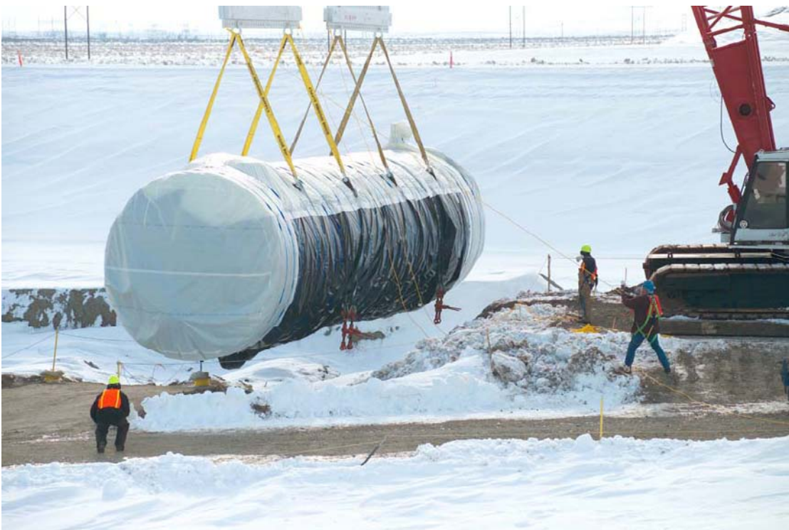
Figure 6-16. Placing PM2A tank from Waste Area Group 1 into the ICDF.
