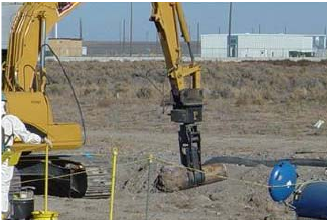
Figure 6-4. Gas cylinder removal at the CPP-84 site.
