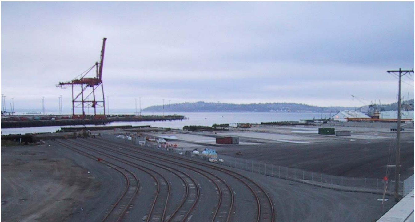
Under the proposed agreement with Lockheed, cleanup of contaminated sediments would begin this summer at the former Lockheed Shipyard on the west side of Harbor Island. (photo courtesy of Hart Crowser)
