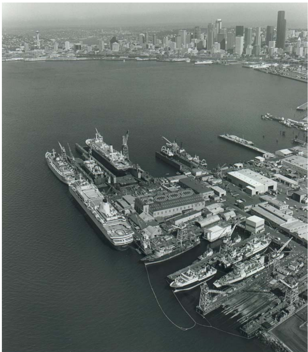
Under the proposed agreement with Todd, cleanup of contaminated sediments would begin this summer at its shipyard on the northwest corner of Harbor Island. (photo courtesy of Floyd Snider McCarthy, Inc.)
