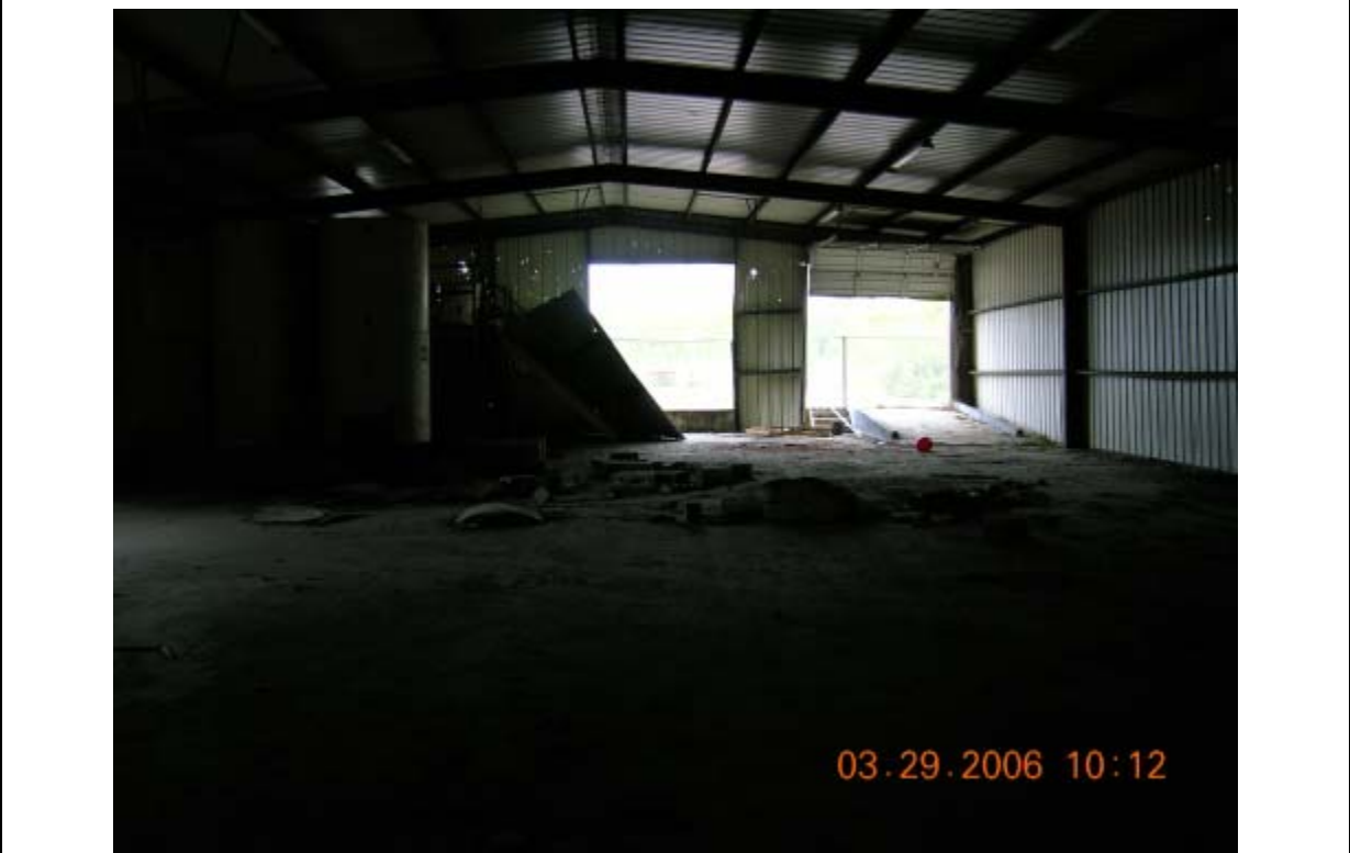
Photo 6: View of inside of Process Building No. 1, facing south. Old debris is lying on the floor inside the building. Doors at the back of the building are fenced to prevent access. These fences are where trespassers have entered the site in the past.
