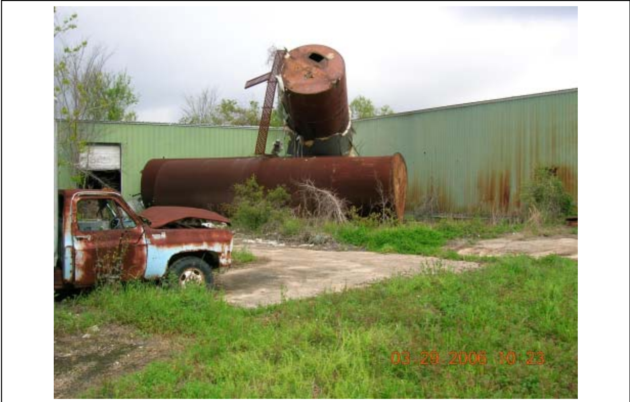
Photo 13: View of site facing northwest, towards corner where Process Building Nos. 1 and 2 join. Old tanks have fallen over.
