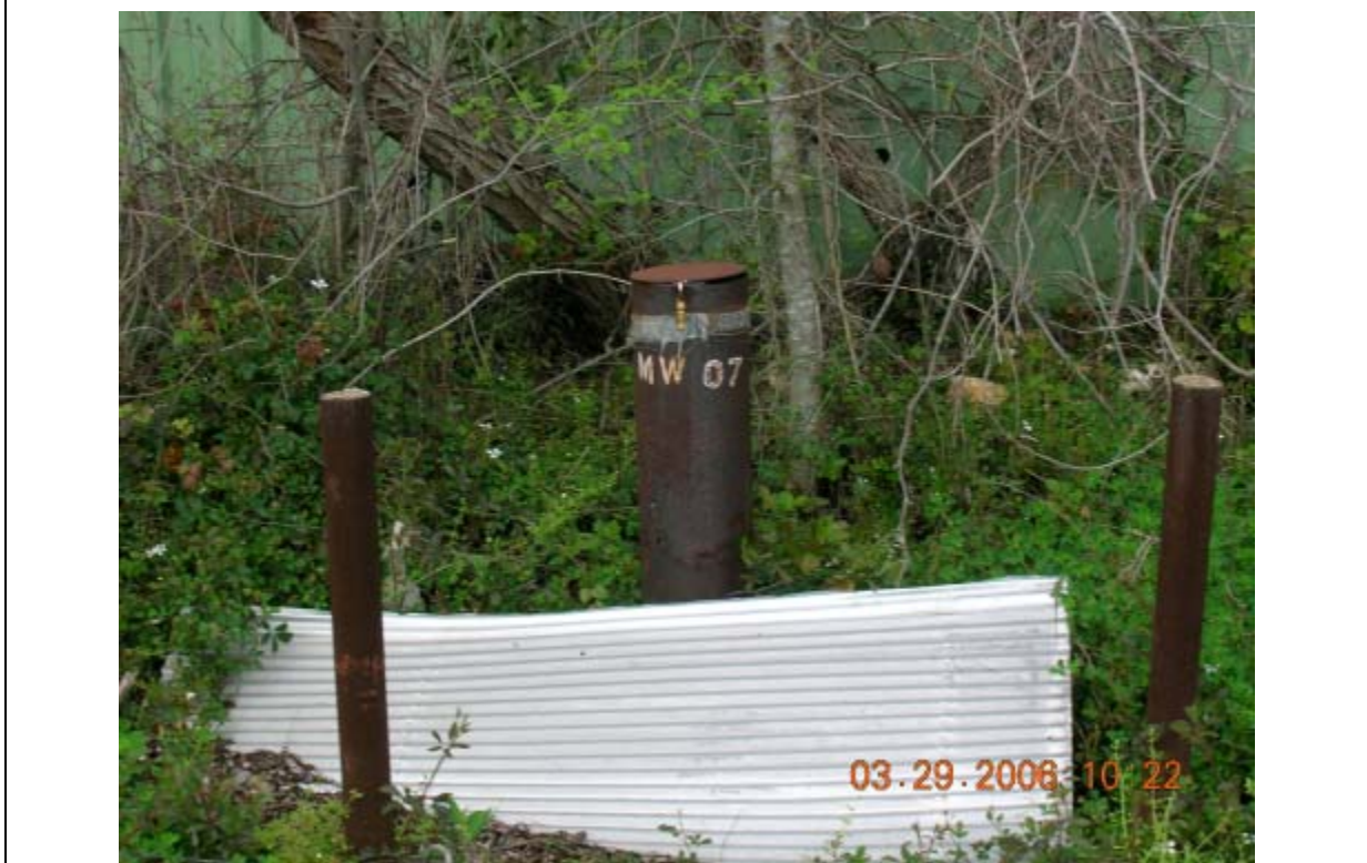
Photo 10: View of monitor well MW-07, located on east side of Process Building No. 1. MW-06 is located north of this well (outside but to the right of this view).
