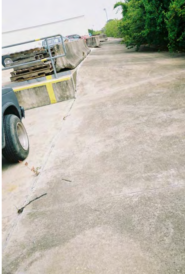
View looking north showing the southeast cap with growth in the joints
