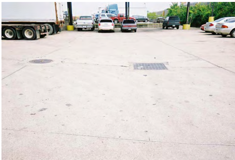
View looking north of southeast cap showing storm drain
