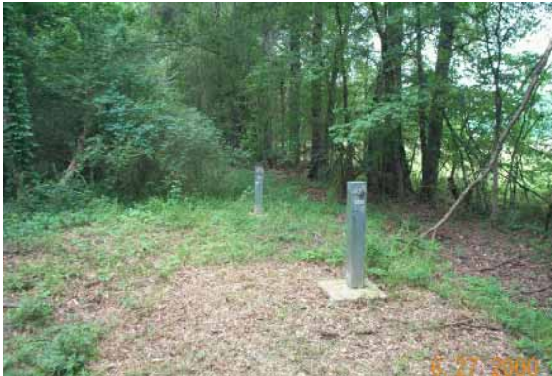
Facing south at south end of Rogers Road. Monitor wells MWR-01 (foreground) and MWR-02 (background). Surface completions appear in good condition.
