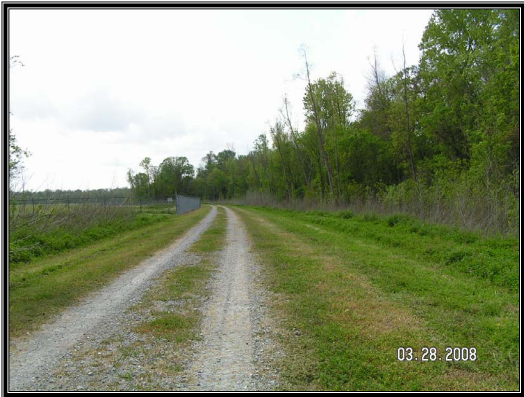
Monitoring Well Pad and Perimeter Road
