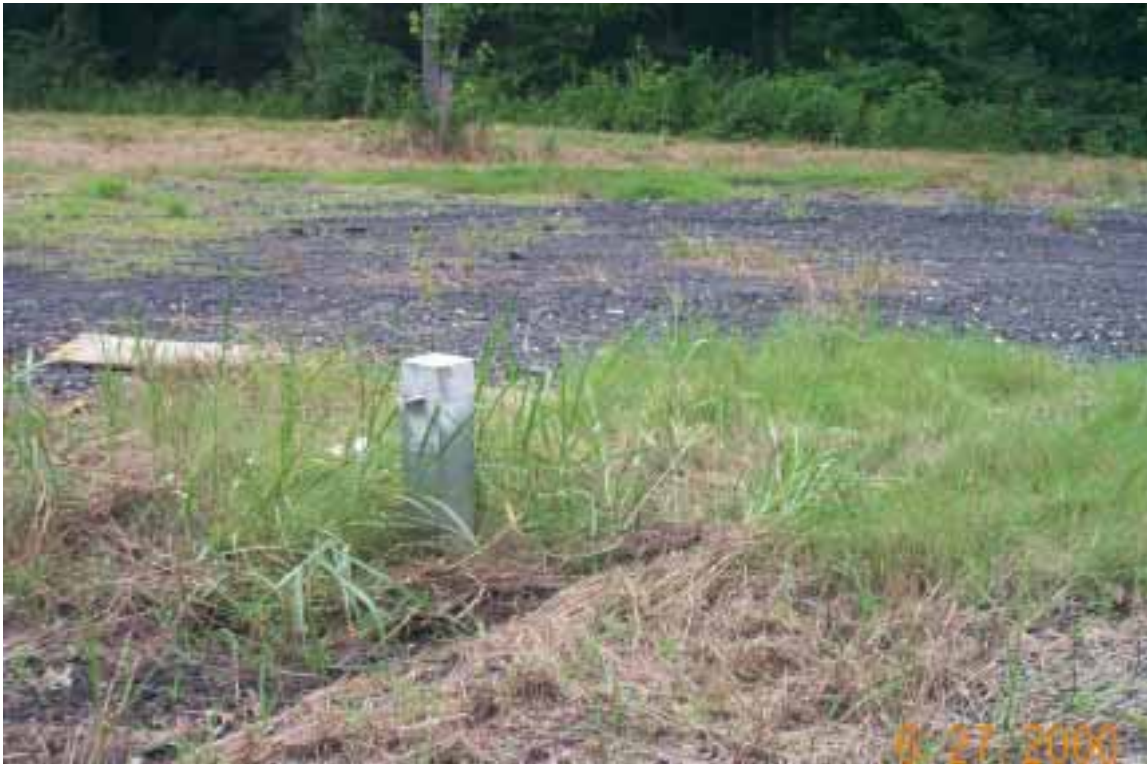
Facing southwest; closeup of monitor well MWJ-13 (also visible in Photographs 10 and 11).
