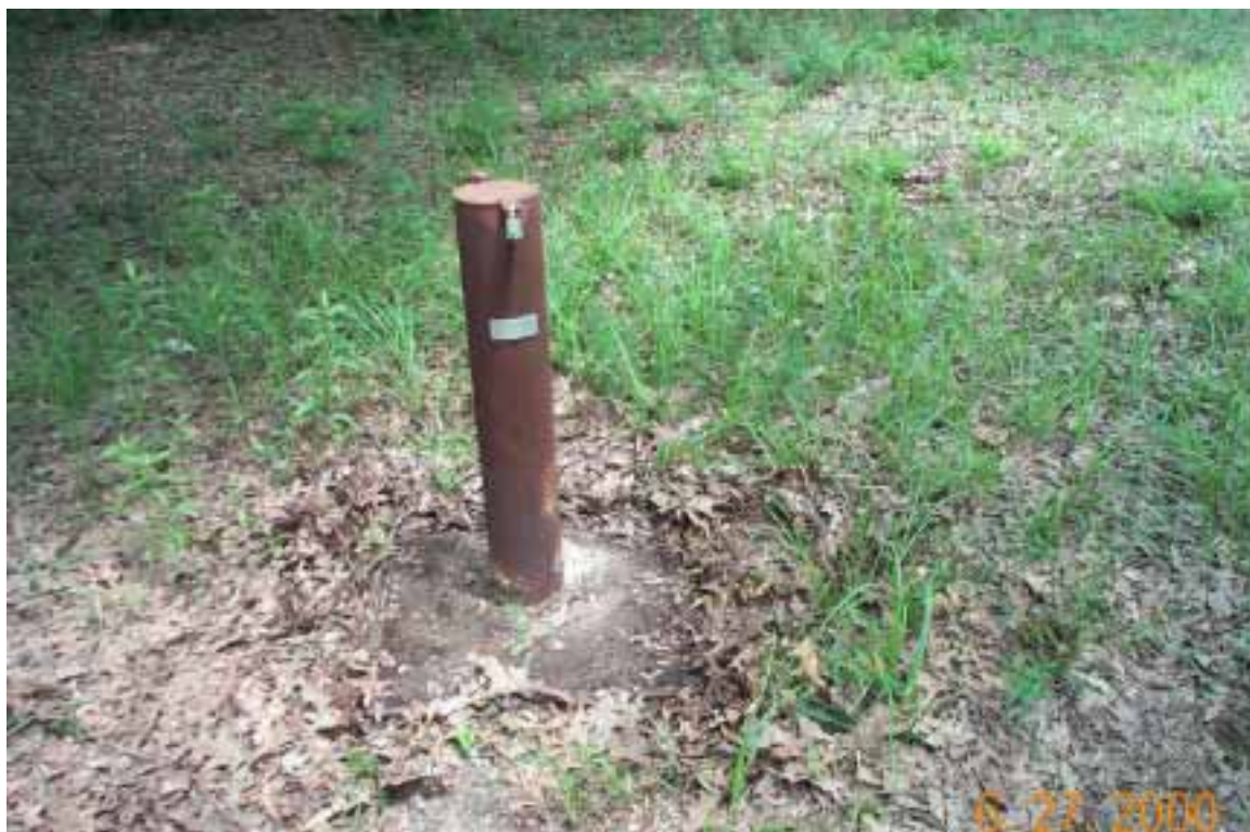
Closeup view of monitor well MWJ-11.
