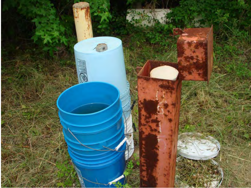
Photograph No. 5 Site: Highlands Acid Pit Superfund Site Description: UA-15 well-missing compression cap, in need of paint, removal of discarded 5-gallon buckets Date: June 20, 2007
