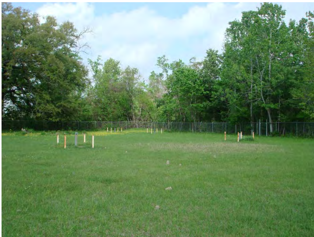
Photograph No. 6 Site: Dutchtown Treatment Plant Superfund Site Description: Northwest portion of site with monitor wells Date: March 29, 2007
