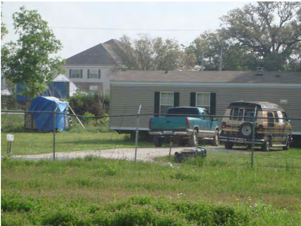
Photograph No. 10 Site: Dutchtown Treatment Plant Superfund Site Description: Damaged fence on east side Date: March 29, 2007 (note residential property developments)
