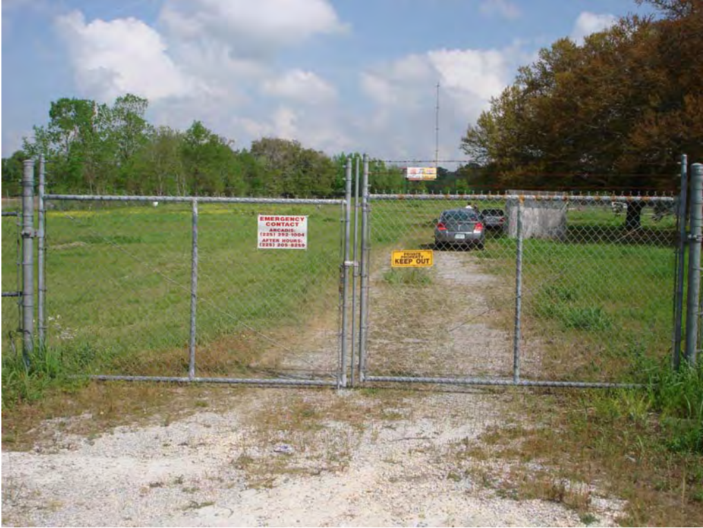
Photograph No. 1 Site: Dutchtown Treatment Plant Superfund Site Description: Entrance gate to site with warning signs Date: March 29, 2007
