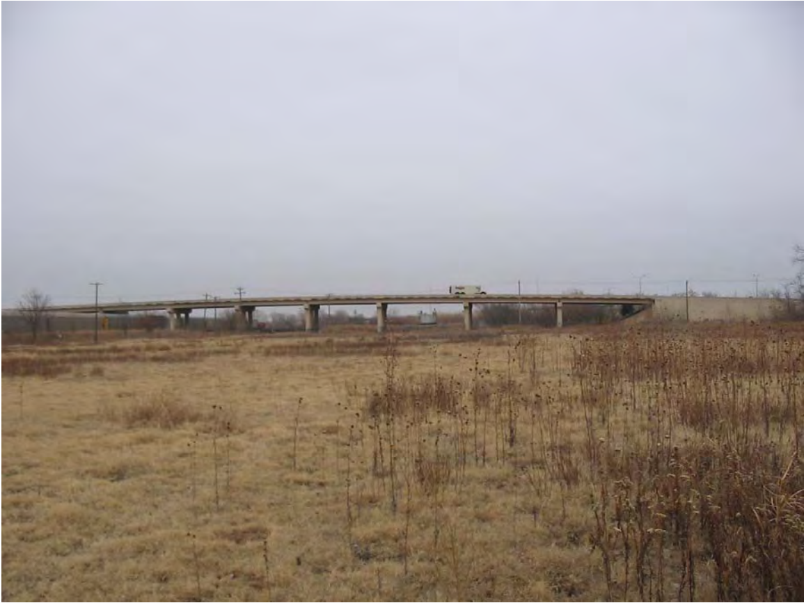
Photo 1: The Double Eagle Superfund site from the west looking towards the east.
