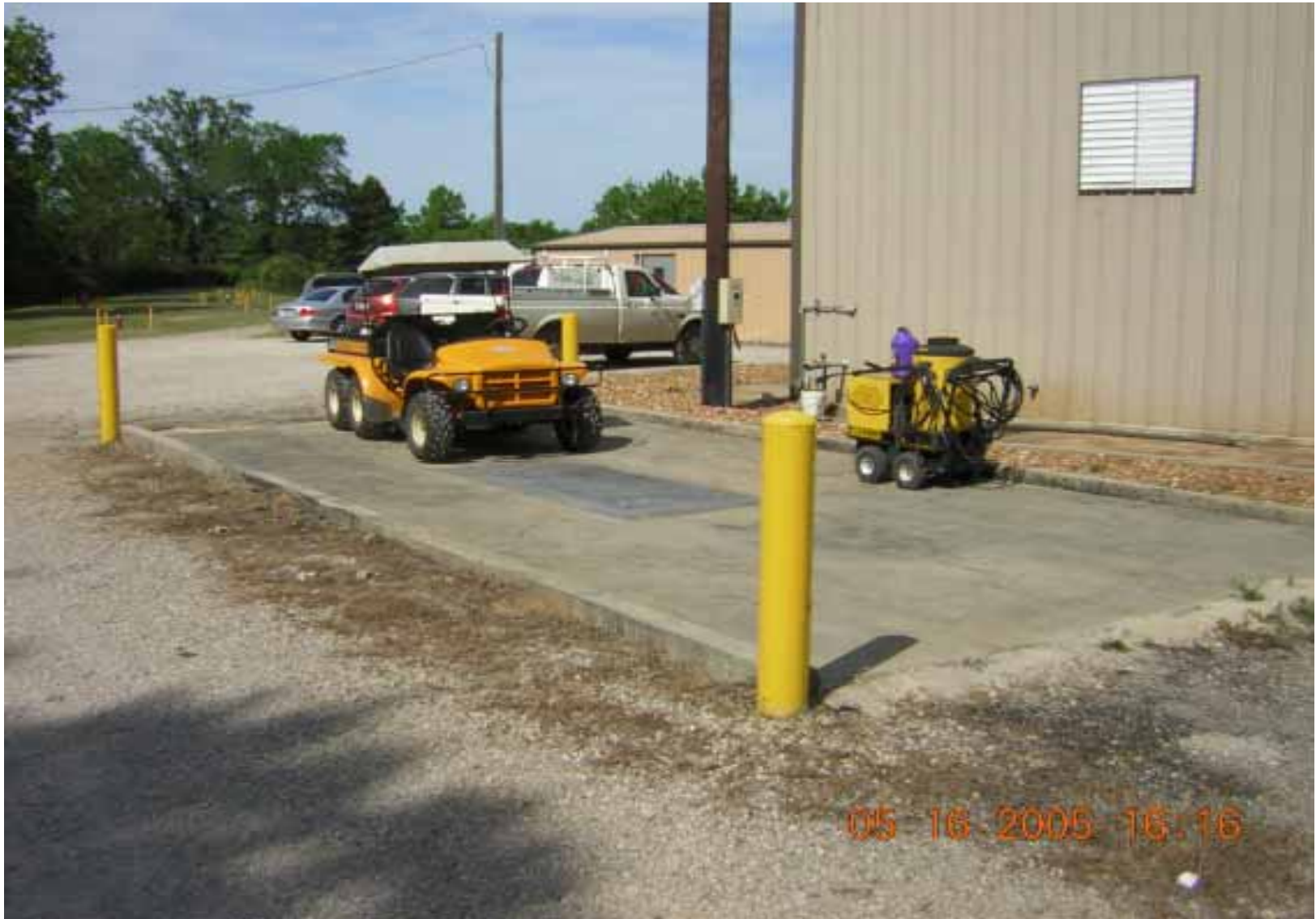
Photo 21: Decon pad located on the west side of the PLTS. This area is not used to change-out the carbon in the carbon filter. Sump in the center of the pad returns fluids to the PLTS.
