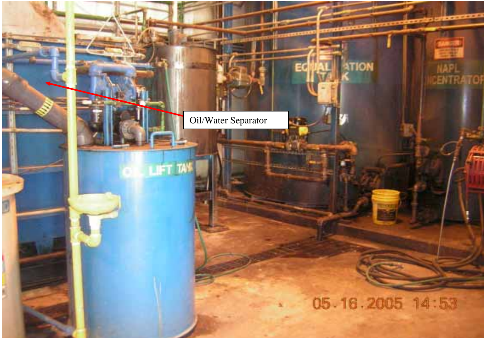
Photo 5: Inside of the PLTS Building. The tank in center background is the equalization tank (used to store water from the well field as it enters the PLTS). To the right of the equalization tank is the NAPL storage tank. The Oil/Water Separator is on the left.
