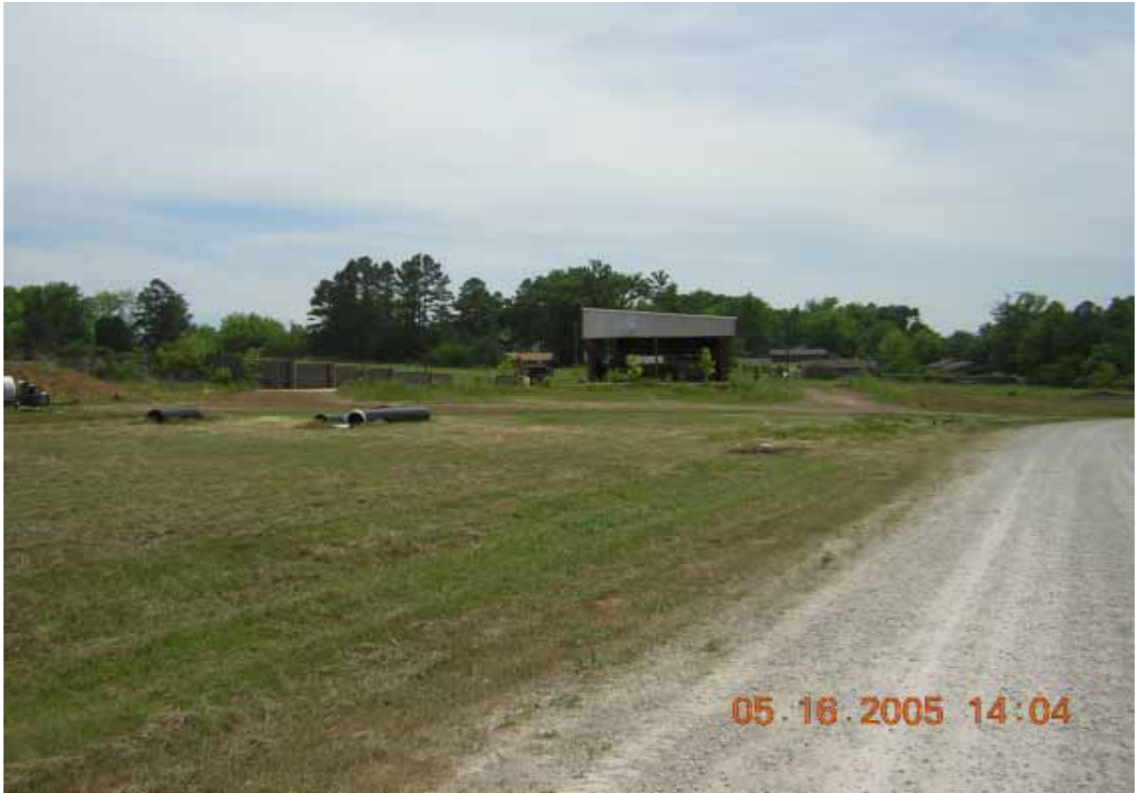
Photo 3: View of south property facing south. Building at center of photograph was used as part of the incinerator operation.
