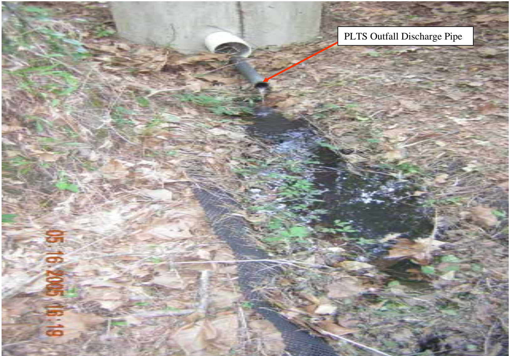
Photo 25: PLTS outfall discharge pipe.
