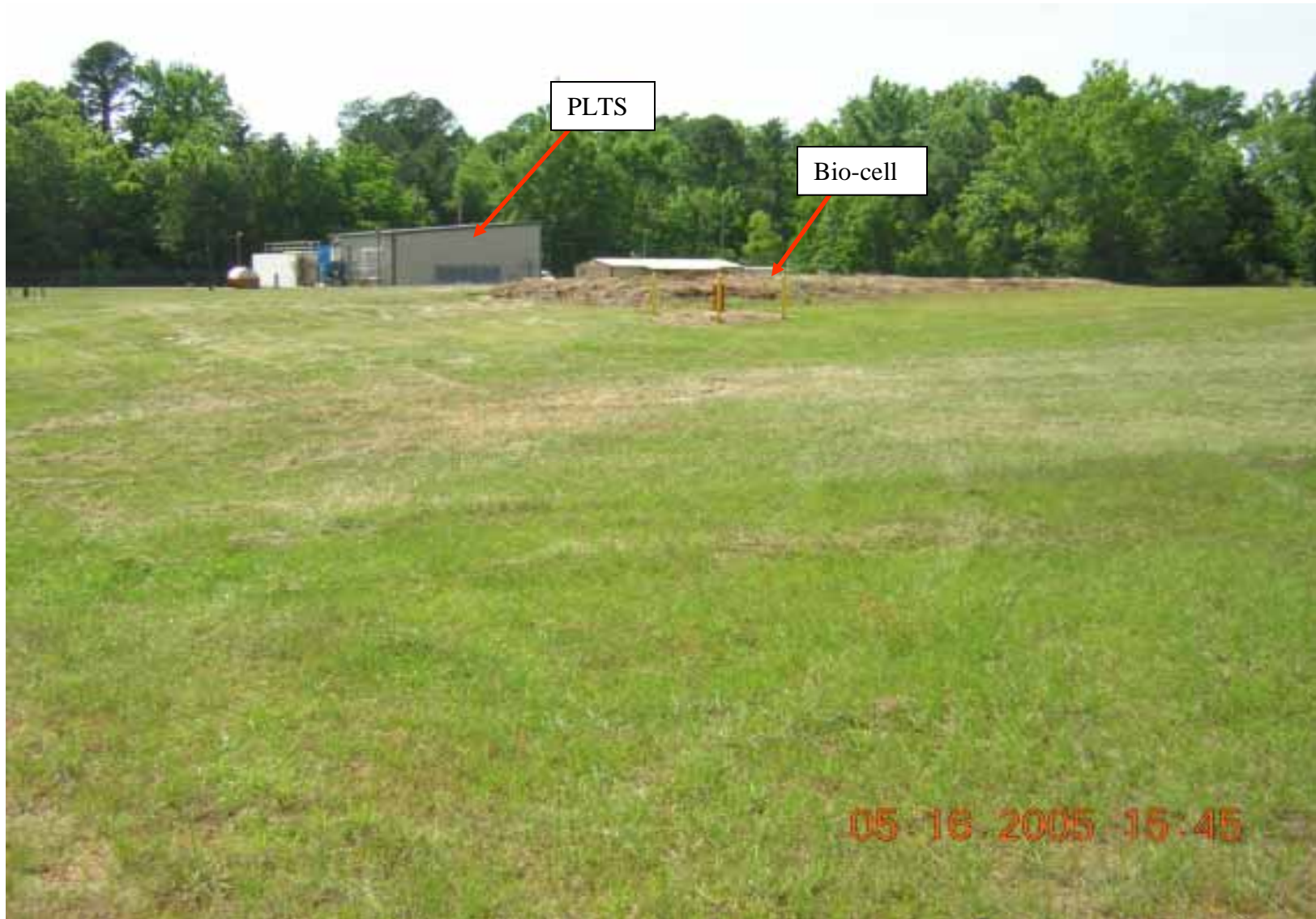
Photo 15: View of the Waste Cell and bio-cell (used to manage bio-solids). The Waste Cell is the grassy area in the center of the photograph. The PLTS is located in the center background.
