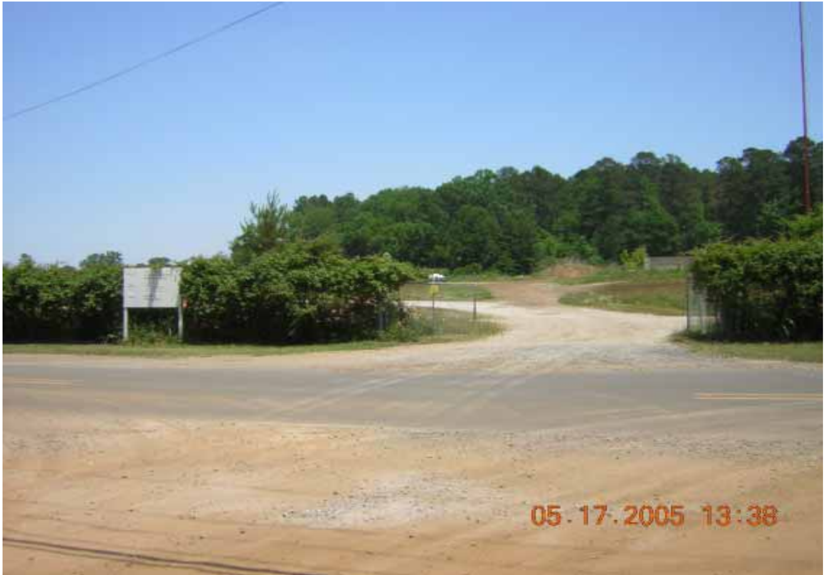
Photo 35: View of front entrance to site, located on Front Street.
