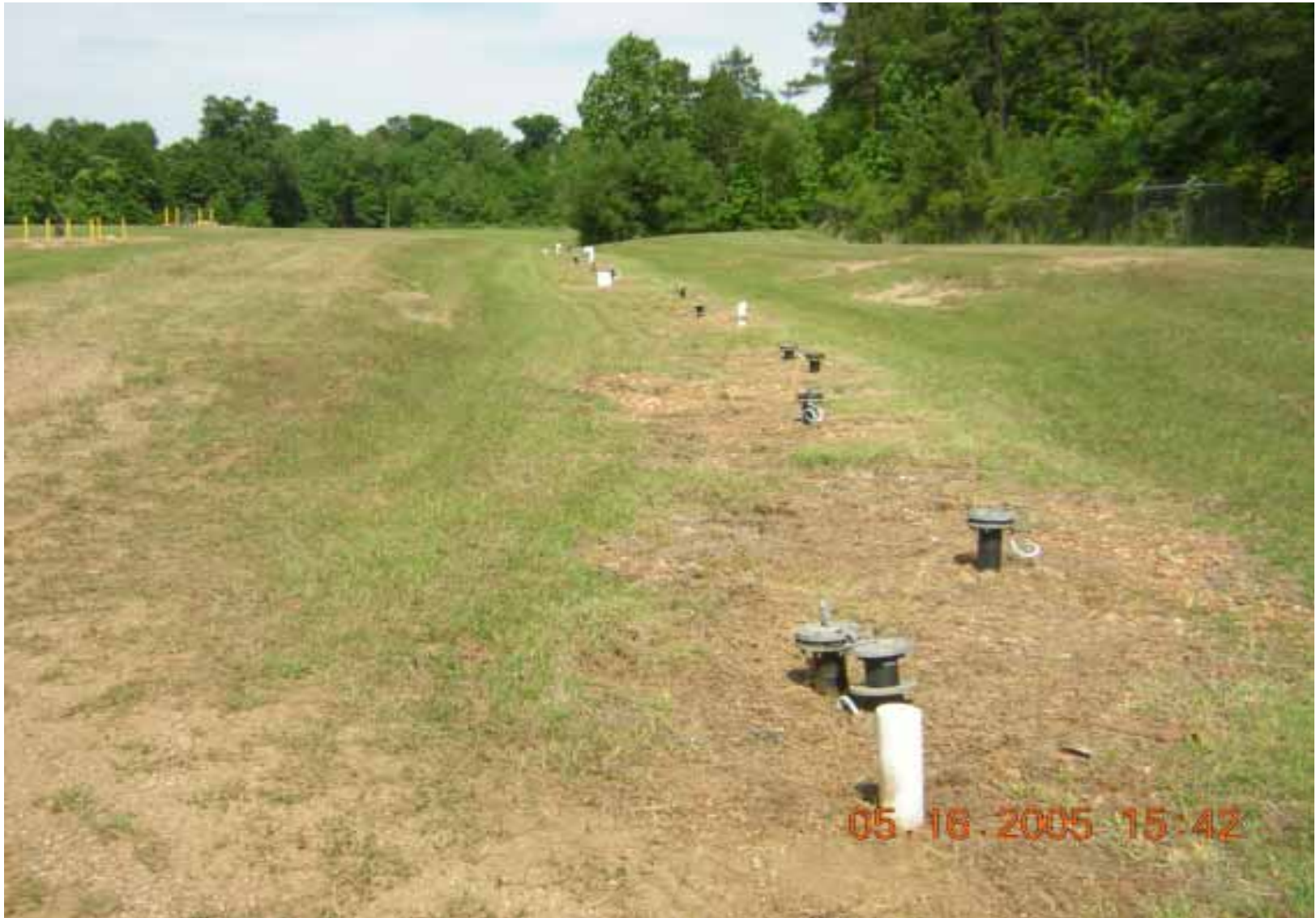
Photo 14: Closer view of the injection trench along its eastern end.
