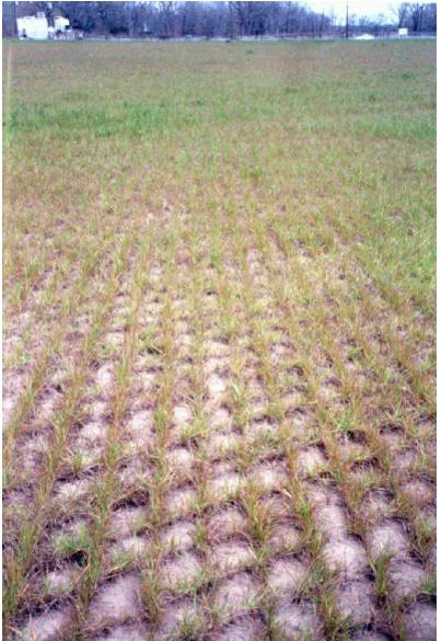
Detail of grass cover (onsite picture, looking east). As part of the remedial action, contaminated soils were removed from the lagoon and waste disposal areas. Soils were treated in the LTU. After treatment soils were backfilled into the former excavation areas. The site was graded to provide adequate drainage, capped with a clay cap, top soil was placed over the cap and the entire site was vegetated with grass.
