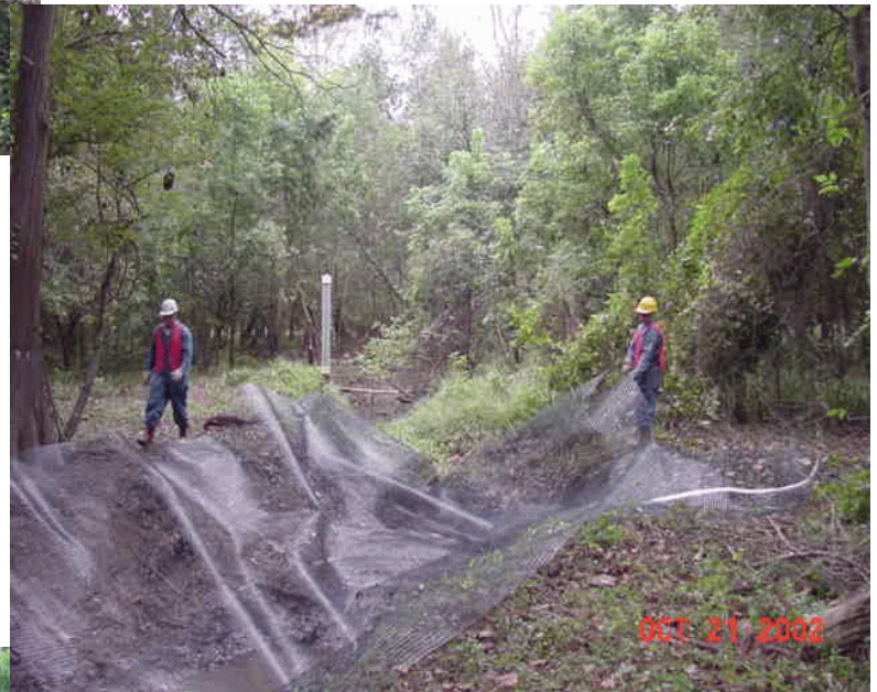
Same section of channel, cleared, with workers installing the liner
