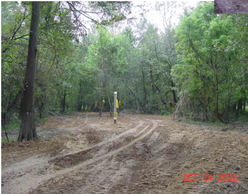
Same section of channel, with backfill activities completed
