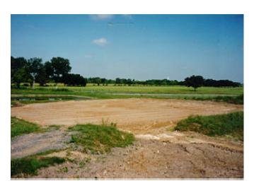
On-site pit where biological treatment residuals and stabilized metal-contaminated material are placed (pit will be capped at end of project)
