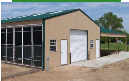
Solar panels will heat and cool the Recycling Center
