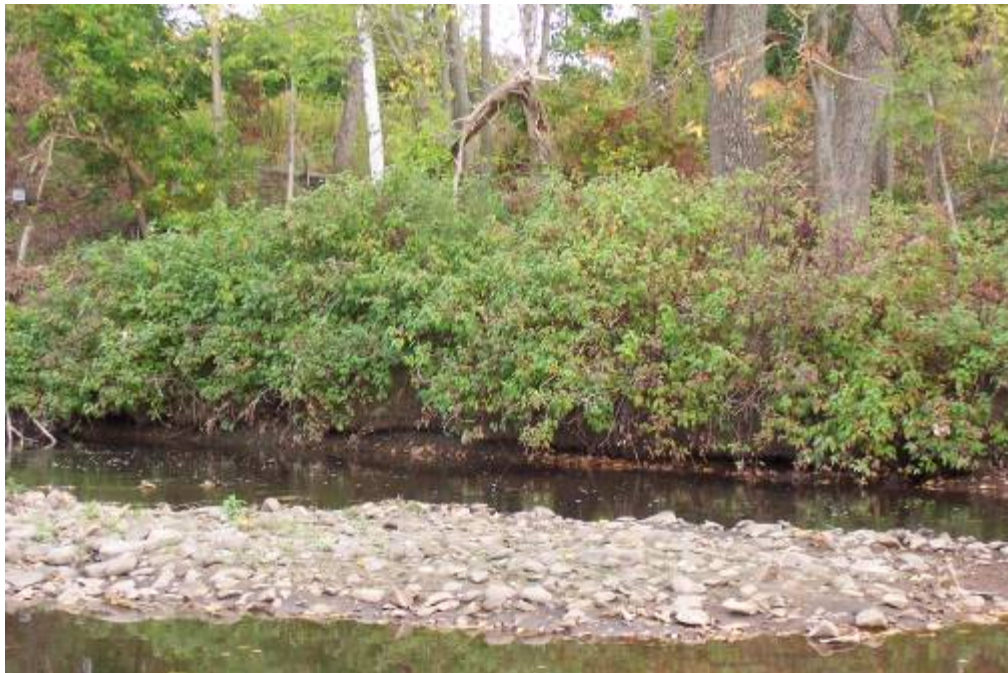
Photo 6 – Area 2A: Approximately 200 ft of undercut bank
