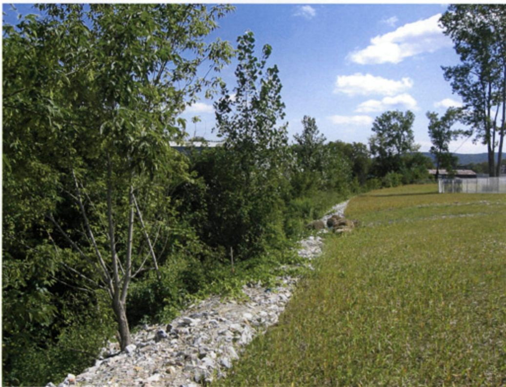
Photograph 7: Planting Area 8, 9, 9A, 11, 11A
