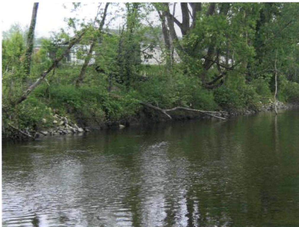
Photo 3 – Area 2: Approximately 100 feet of slight undercut downstream of swale.
