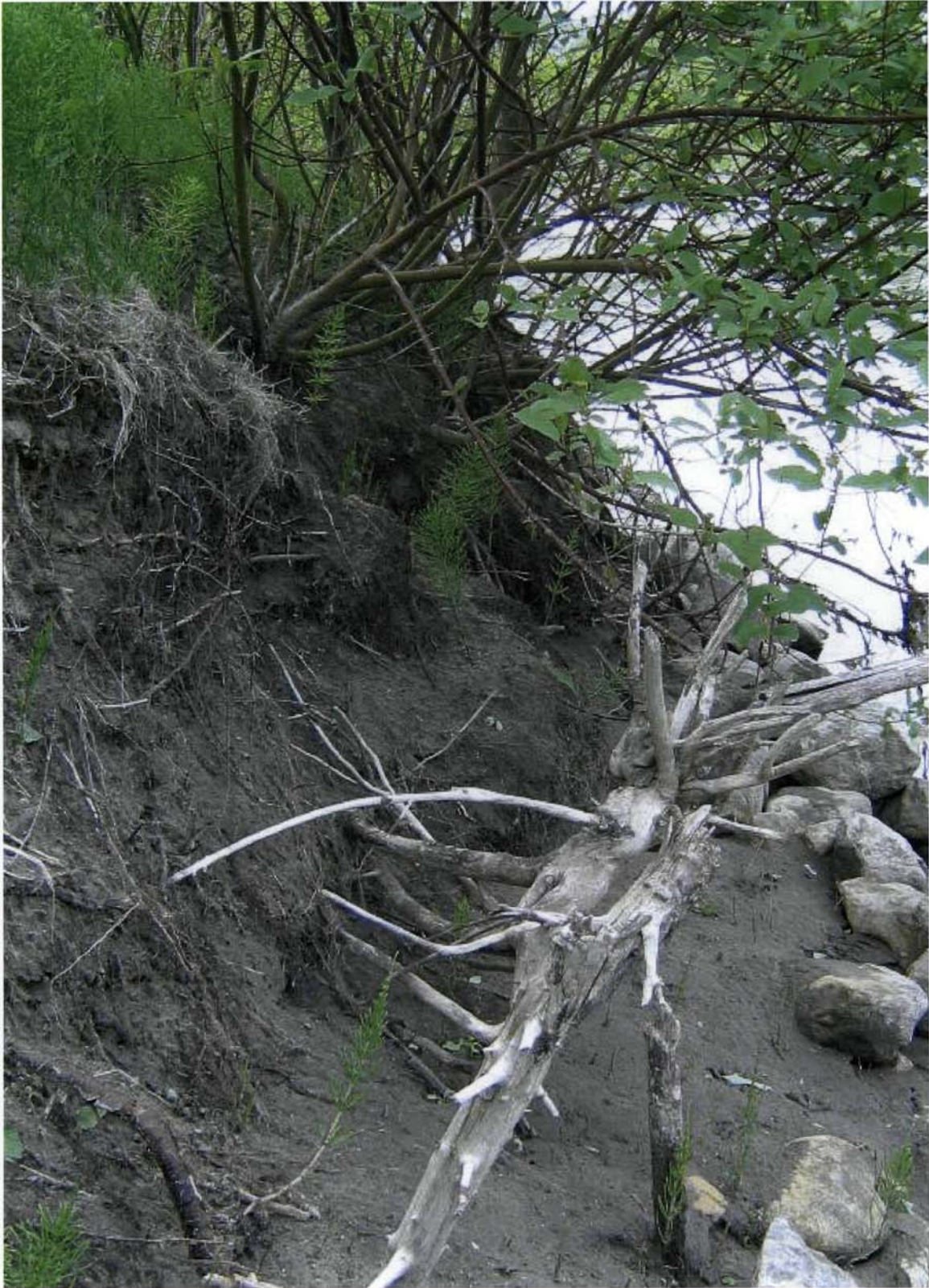
Photo 7 – Area 5: Example of near vertical face proposed for removal.
