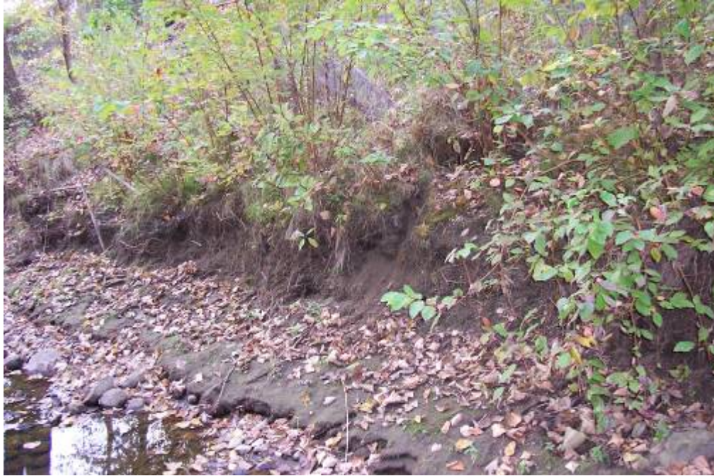
Photo 1 – Area 1A: Undercut bank
