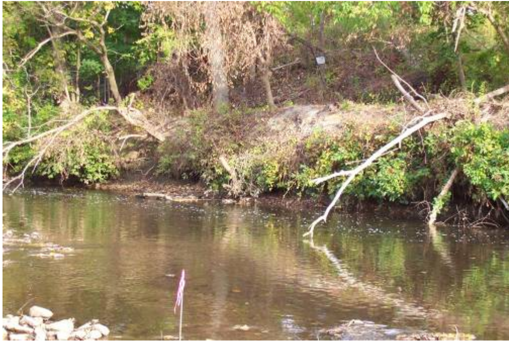
Photo 5 – Area 2A: Approximately 200 ft of undercut bank
